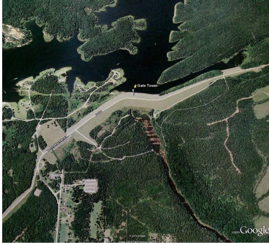
Figure 3. Aerial View of Embankment and Outlet Structure
