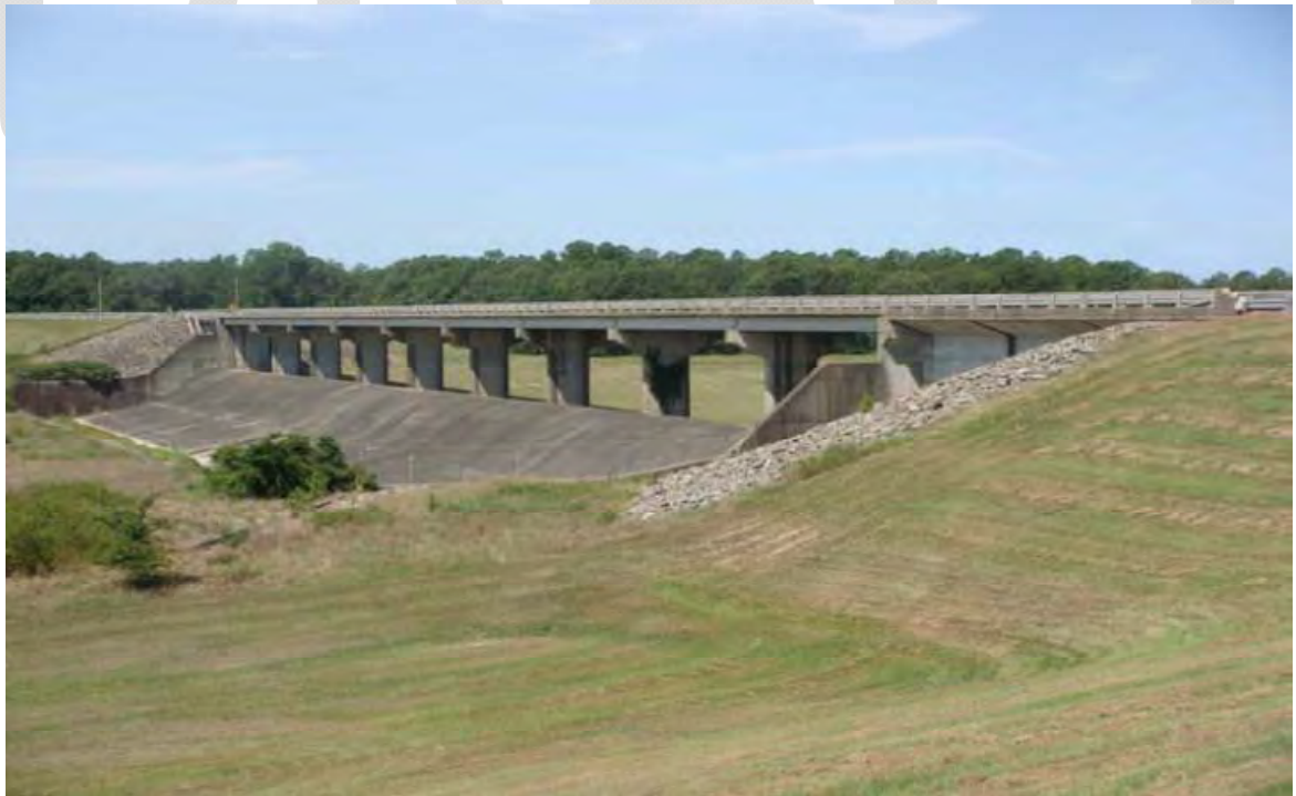
Figure 1.4. Uncontrolled spillway.
