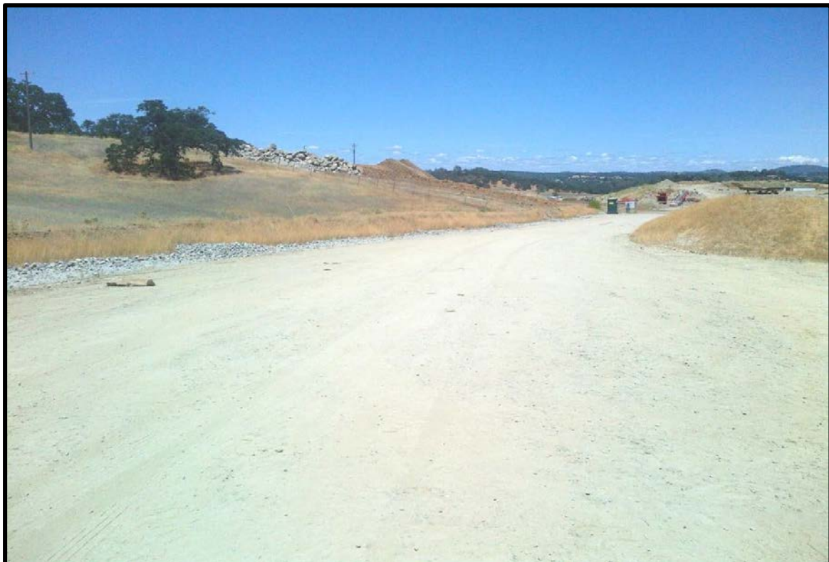
Photo 2. Interior haul road. View from ground level.
