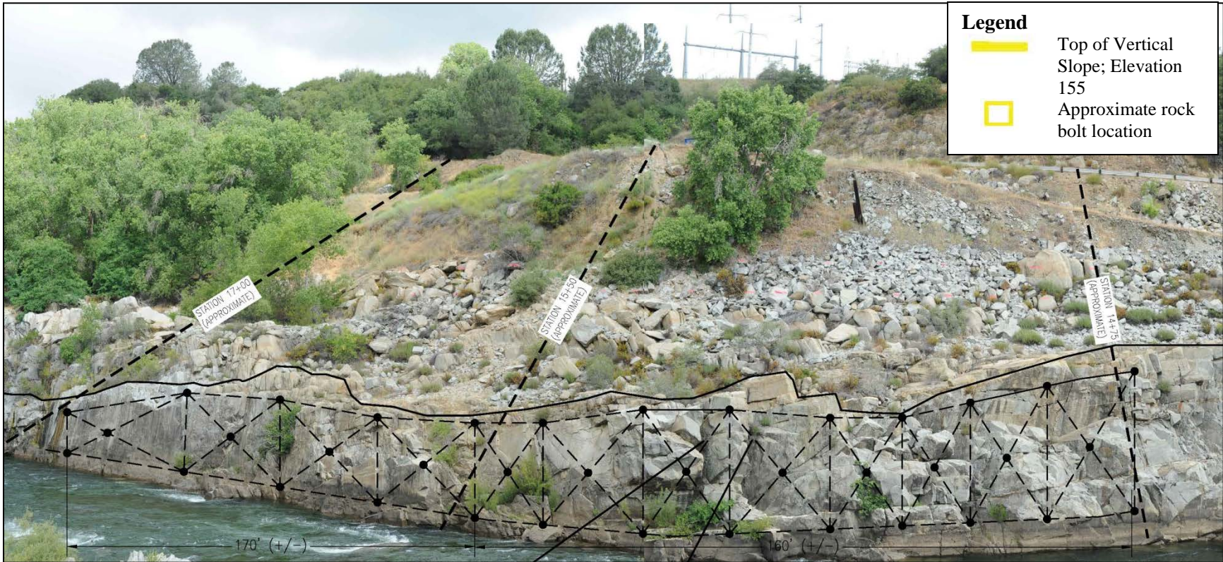
Figure 3. Approximate Rock Bolt Locations
