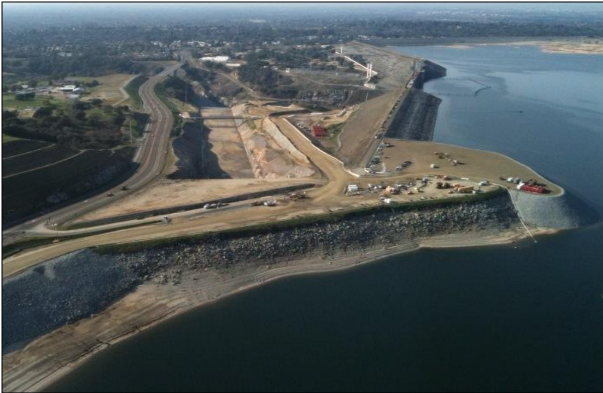
Figure 11. Aerial View of Shoreline at Approach Channel and Folsom Overlook.
