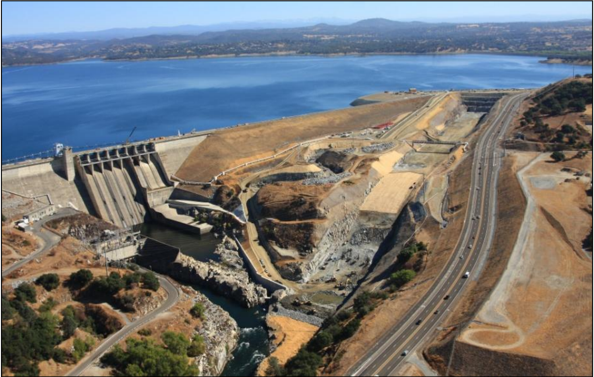
Figure ES-4. Aerial View of Project Area and Folsom Dam.
