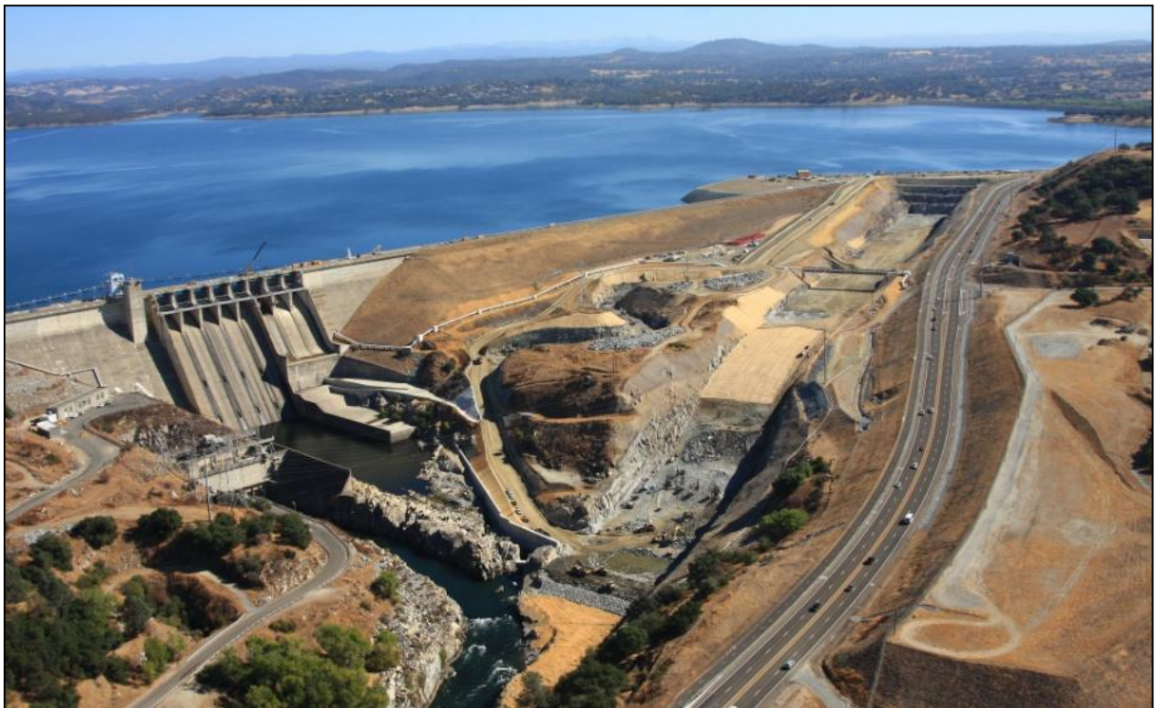
Figure 10. Aerial View of Project Area and Folsom Dam.
