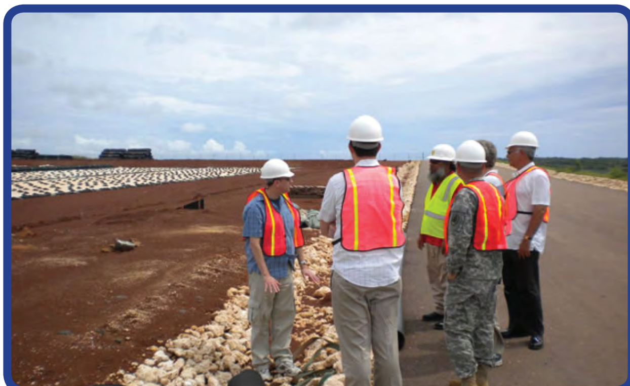
DoD OIG team inspecting the new solid waste facility in Guam.
