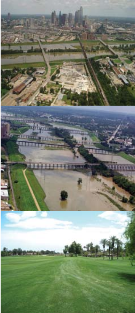
Top Two Photos: Levee in major urban area. Dallas, TX— Courtesy of City of Dallas Flood Control District
