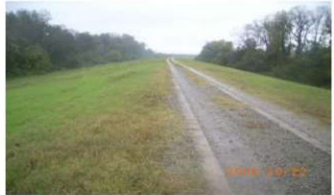
Lower Arkansas River, South Bank Levee
