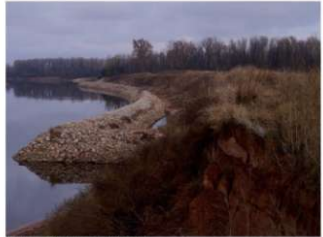
Dickson Revetment Phase I
