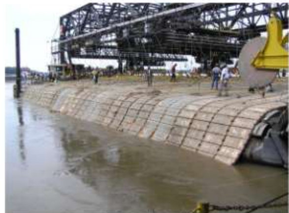
Revetment Construction – Articulated Concrete Mat (ACM)
