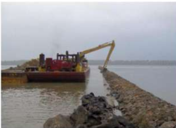
Stone Dike Construction
