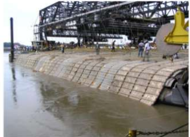
Revetment – Articulated Concrete Mat
