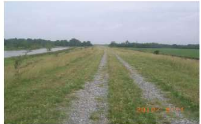
Lower Arkansas River, North Bank Levee
