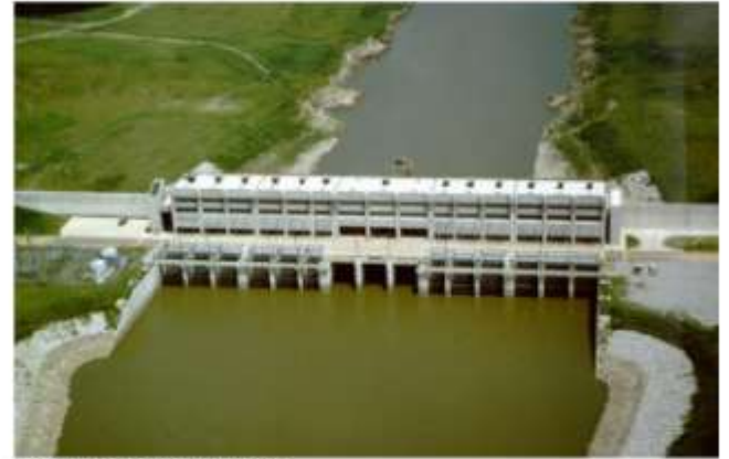
Lake Chicot Pump Plant
