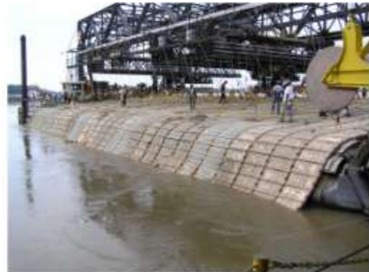
Revetment Construction – Articulated Concrete Mat (ACM)
