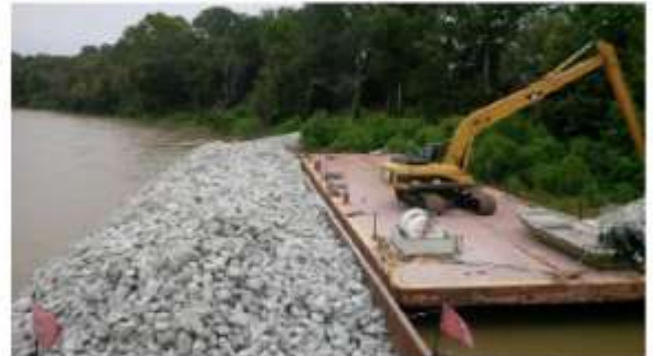
Figure 1. OD-RC equipment performing similar work in a small river environment
