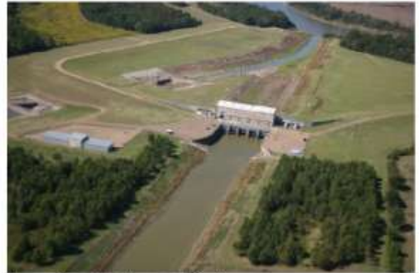
Tensas-Cocodrie Pumping Plant
