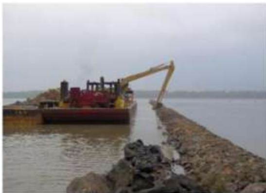
Stone Dike Construction
