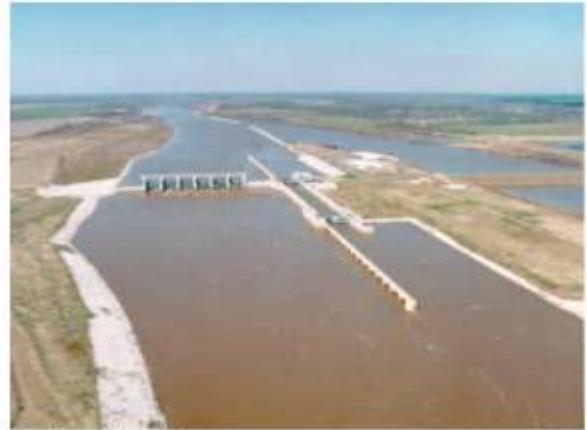
Lock and Dam #3
