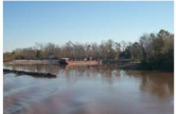
Figure 1. Similar Repairs on the JBJWW
