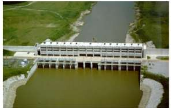
Lake Chicot Pump Plant
