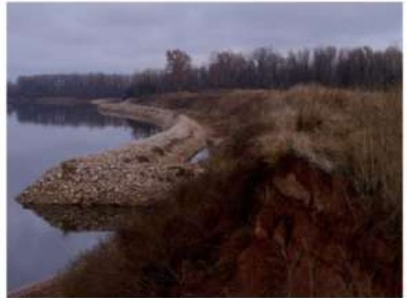
Dickson Revetment Phase I
