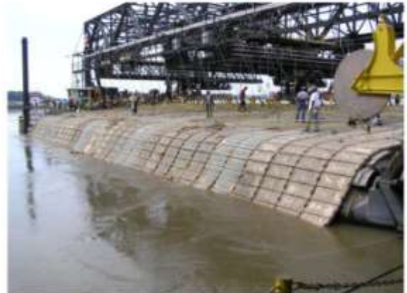
Revetment – Articulated Concrete Mat
