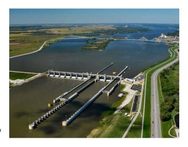
The complex has twin locks. The main lock is 110 by 1,200 feet; the auxiliary lock is 100 feet by 600 feet. The locks are U-shaped and supported on steel H-piles. The maximum lift is 24 feet.
