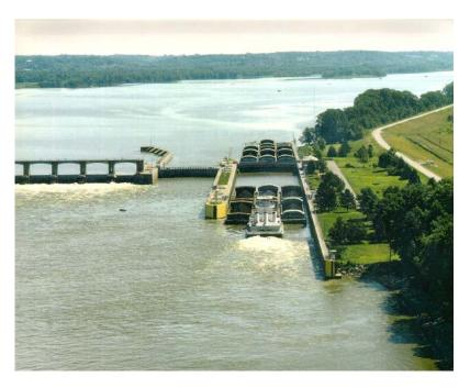
The movable dam has 12 non-submersible Tainter gates (20 feet high and 40 feet long), three submersible Tainter gates of the same dimensions, and four non-submersible roller gates (20 feet high and 80 feet long). The dam system also includes a linear, concrete capped, ogee spillway; and a submersible earth and sand-filled dike. It takes eight hours for water to travel from Lock and Dam 15, in Davenport, lowa, to Lock and Dam 16.
