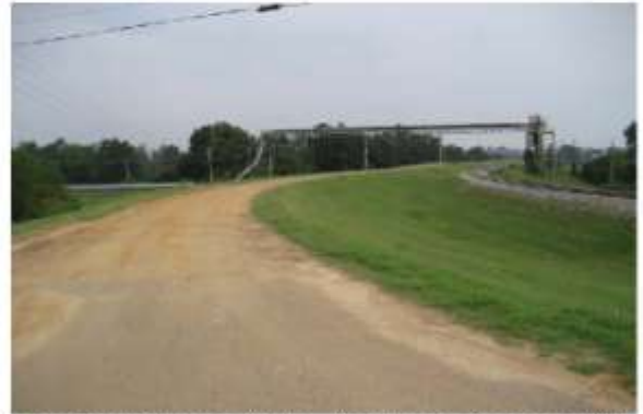
Yazoo City Protection Works - East Levee - Station 44+00
