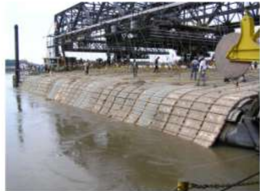
Revetment Construction – Articulated Concrete Mat (ACM)
