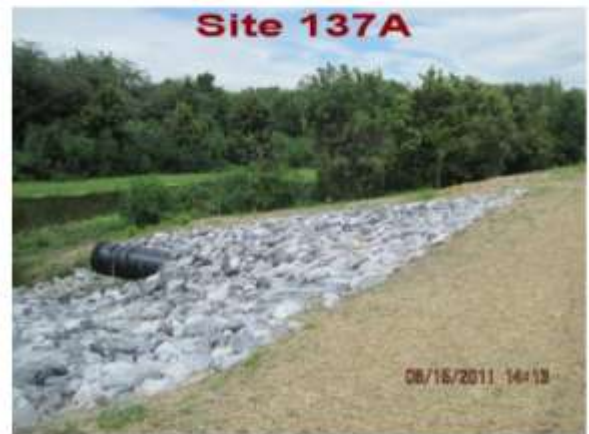
Sediment Reduction Structure
