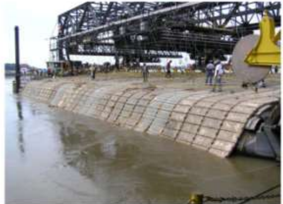
Revetment – Articulated Concrete Mat
