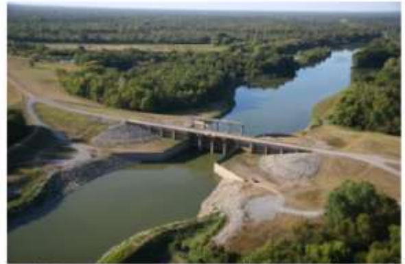
Steele Bayou Drainage Structure on the Yazoo Backwater Levee
