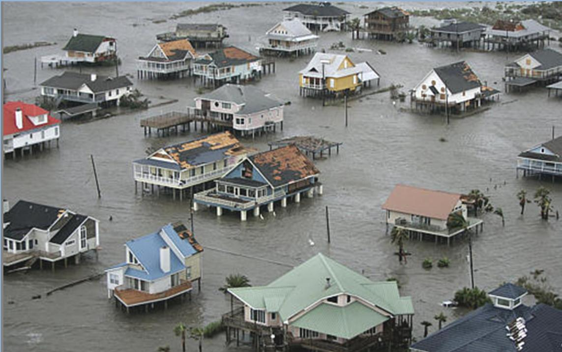
The elevated homes in the picture above appear to have only wind-related damages. If these homes were constructed at-grade, the inundation alone would have caused significant damage or total destruction.
