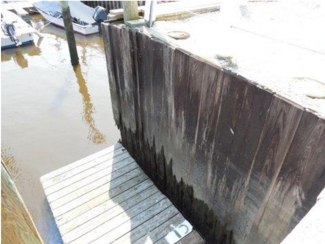
Existing Bulkhead along Bay Avenue
