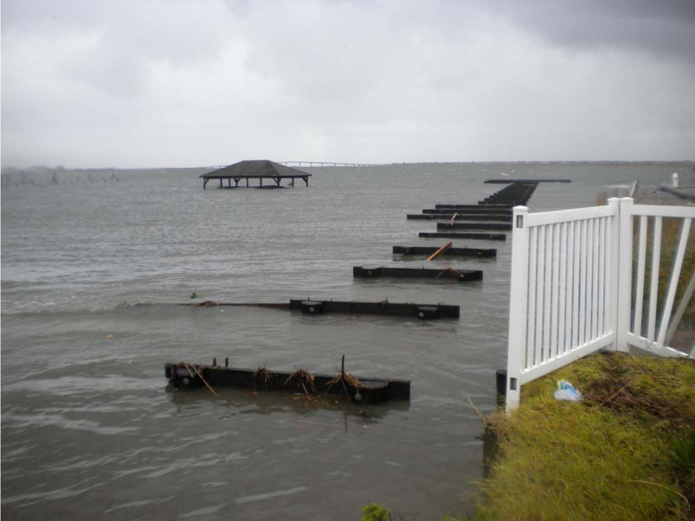
Fishing Pier and Gazebo destroyed by Sandy
