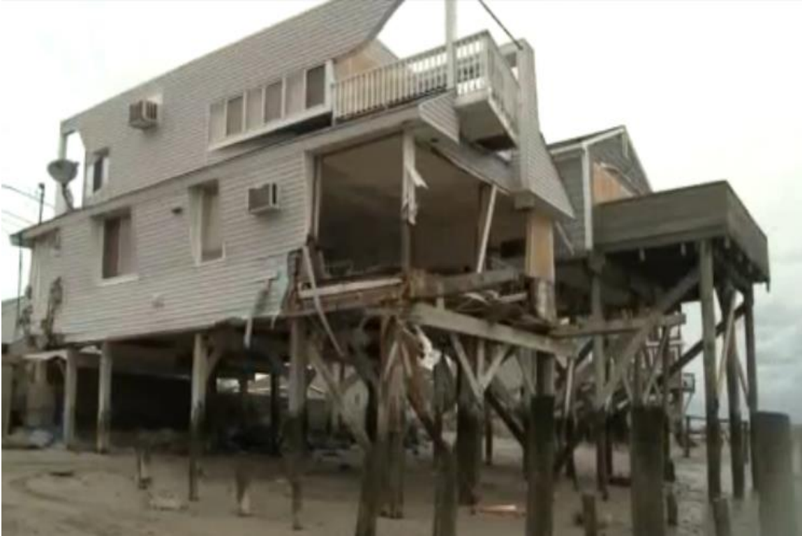
Figure 11. Fairfield Beach Road
