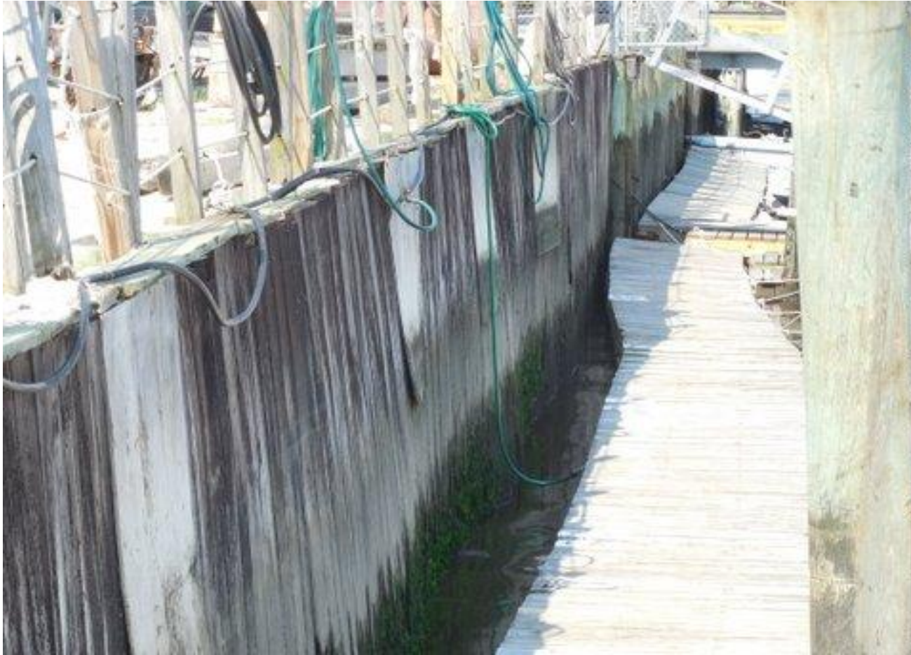
Existing Bulkhead along Bay Avenue
