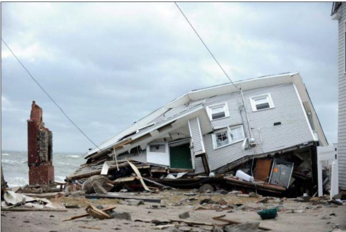
Figure 12. Fairfield Beach Road
