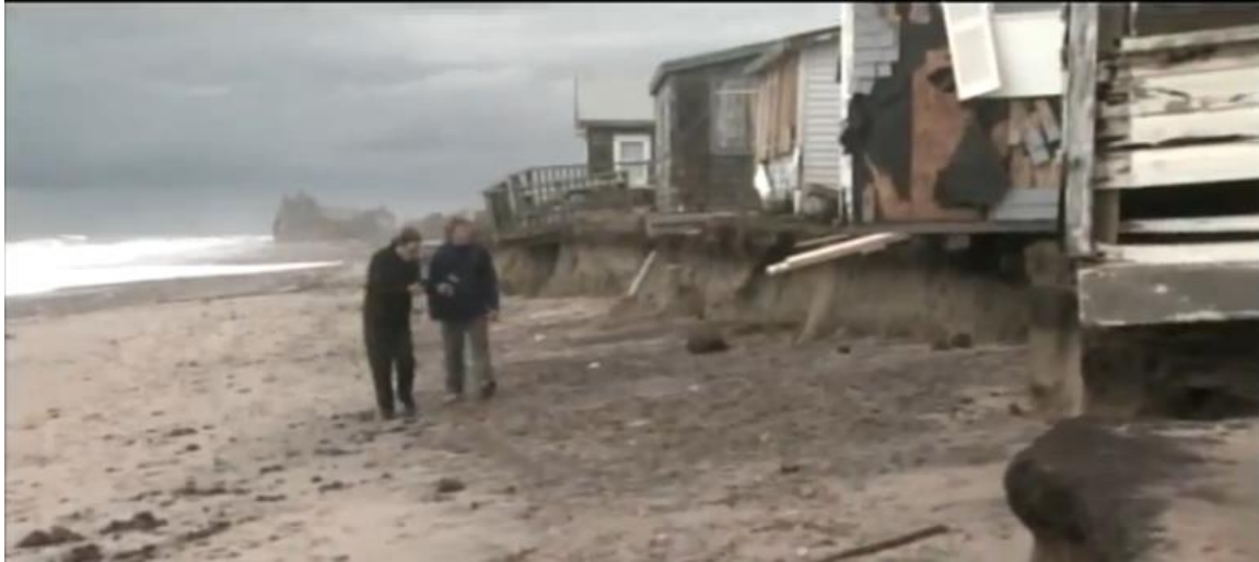
Figure 7. South Kingstown Houses, which had decks and 20-30 feet of grass in their yard prior to Sandy erosion
