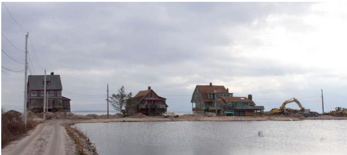
Figure 8. Three Historic Victorian houses on Browning Beach were so badly damaged that they had to be destroyed (Providence Journal Photo)
