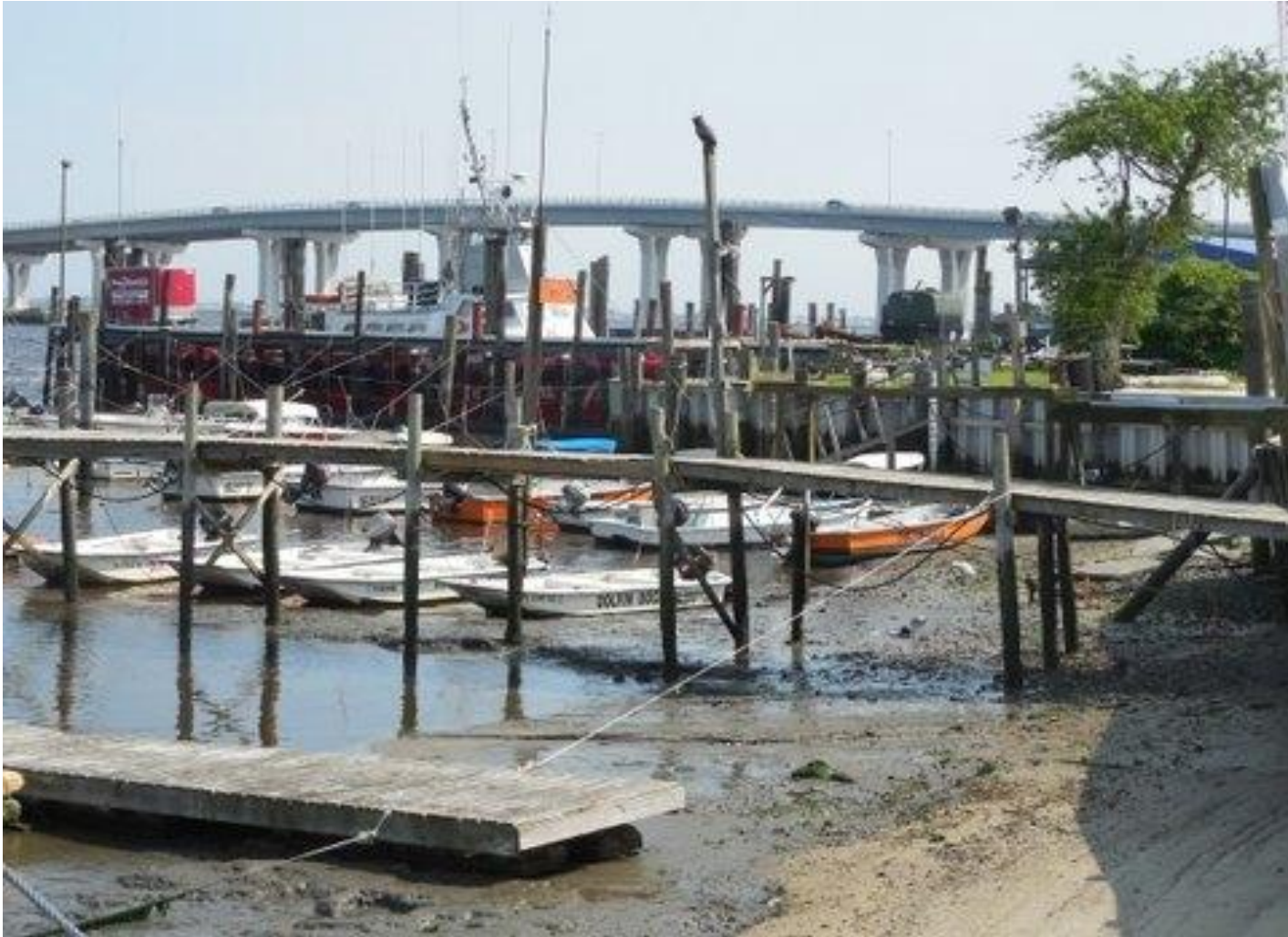
Extremely shallow water at low tide along Bay Avenue
