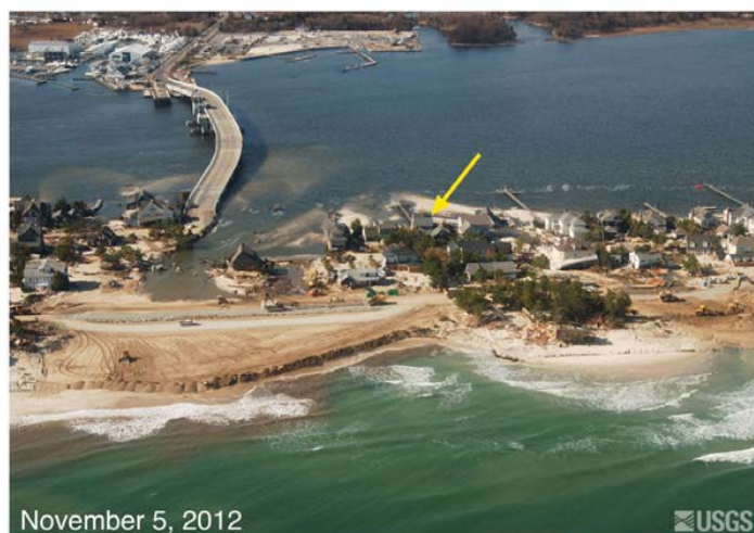
Figure III-13. Before and After Images of a Portion of the Coast in Mantoloking, NJ. Photo Courtesy: USGS
