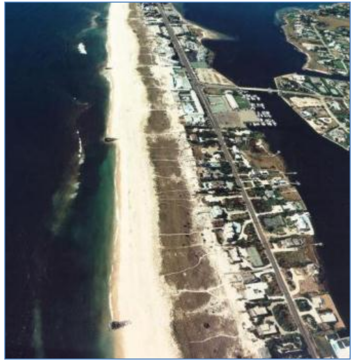
Figure VIII-16. Groin Field at Westhampton, NY
