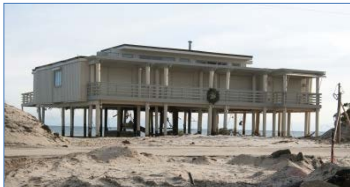
Figure VIII-2. Typical Elevated Shorefront Structure (Courtesy: FEMA)
