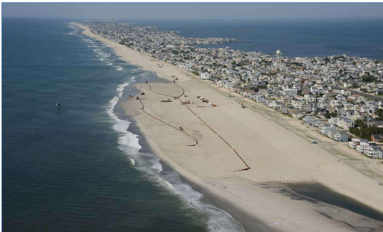
Figure VIII-14. Beach Restoration project under construction in June 2013 at Brant Beach, NJ
