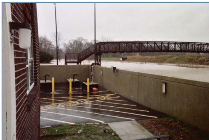
Figure VIII-3. Typical Apartment Ringwall
