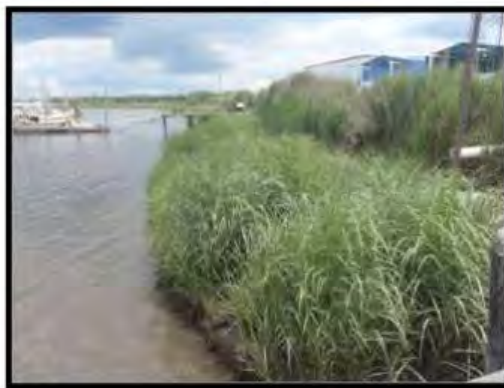
AFTER: One year later, June 2011, native marsh grass can be seen flourishing in the soil that has collected behind the new "living shoreline." Not only does this defend land against destructive waves, but also it serves as fish habitat during high tides.
