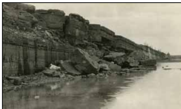
USACE Photo The bottom of the Livingstone Channel, dewatered in this 1933 photo, features formidable bedrock and limestone formations.
