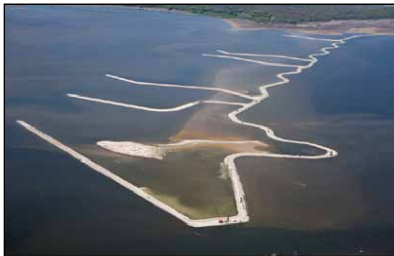
USACE Photo An aerial shot of the Cat Island wave barrier and ‘legs’ that will enclose dredged materials reveals remnants of the original Cat Island in the lower cell.
