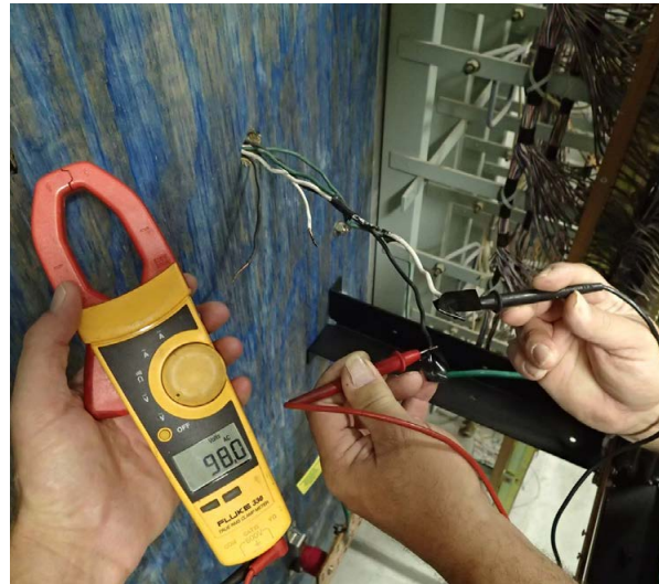
DoD IG inspected military housing facilities in Japan for compliance with applicable DoD and Federal standards.
