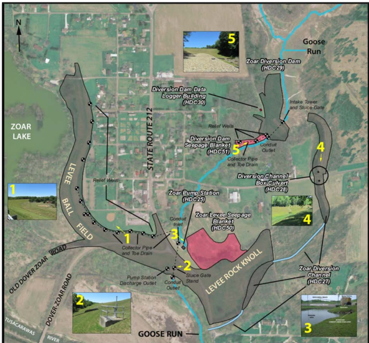
Figure 1-6 Aerial photograph charting major project features of Zoar Levee & Diversion Dam.
