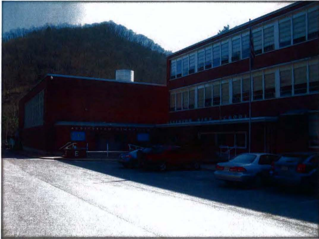
Ervinton High School: Structure OPF-0036; Tract No. 2201
