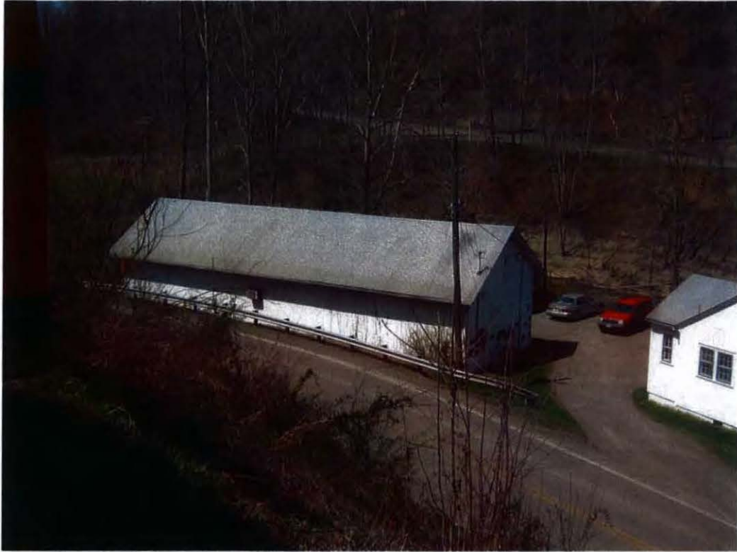
Haysi High School Band/Music Building: Structure RUF-0078; Tract No. 201
