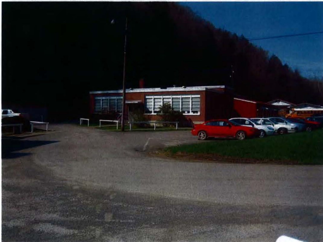
Ervinton High School Technology Center: Structure OPF-0039; Tract 2201
