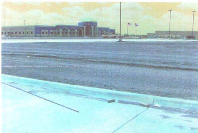
New county jail under construction, west of and adjacent to the site.
