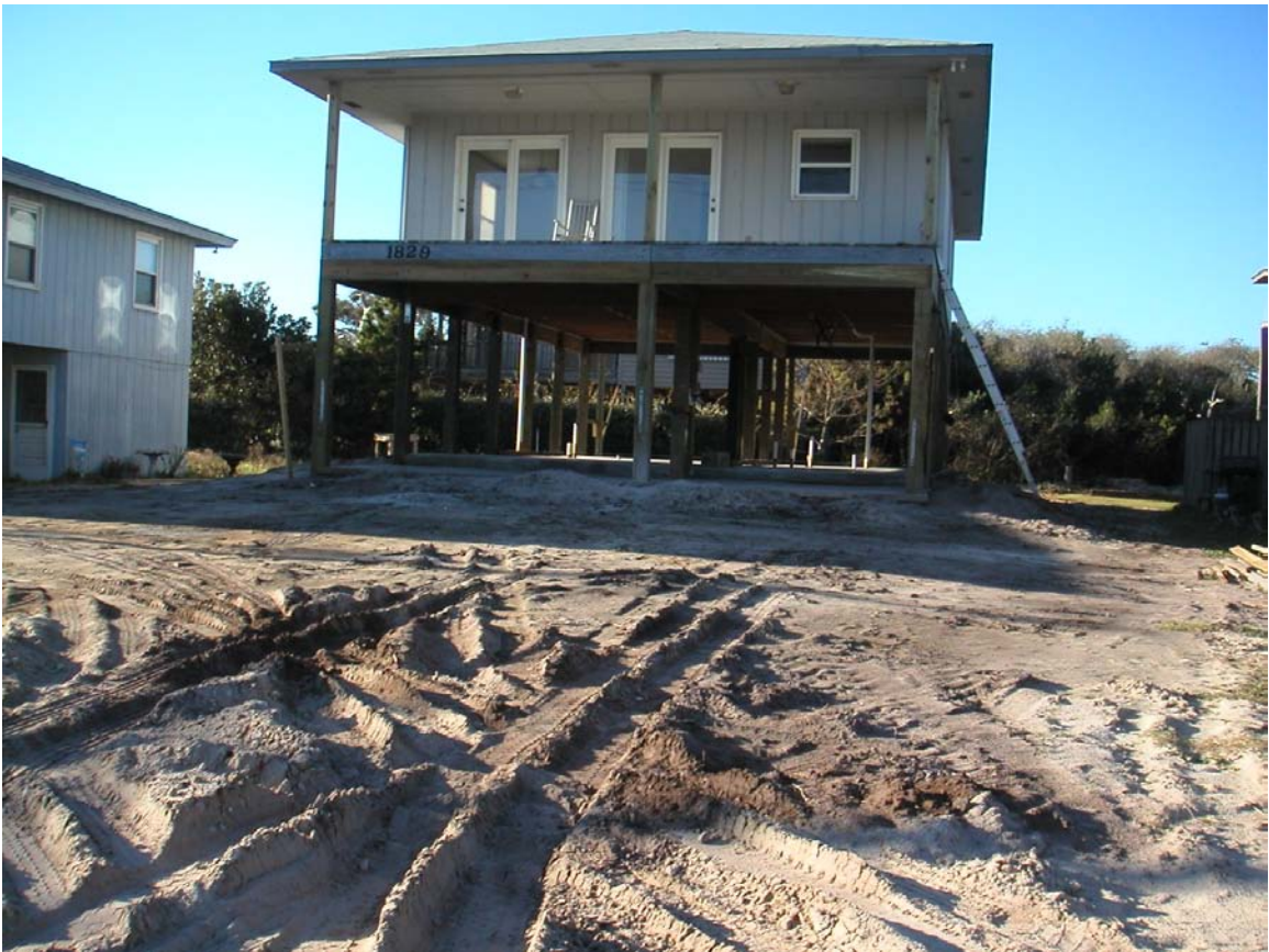
Figure B- 20 Topsail Island home raised on piling foundation 2004.
