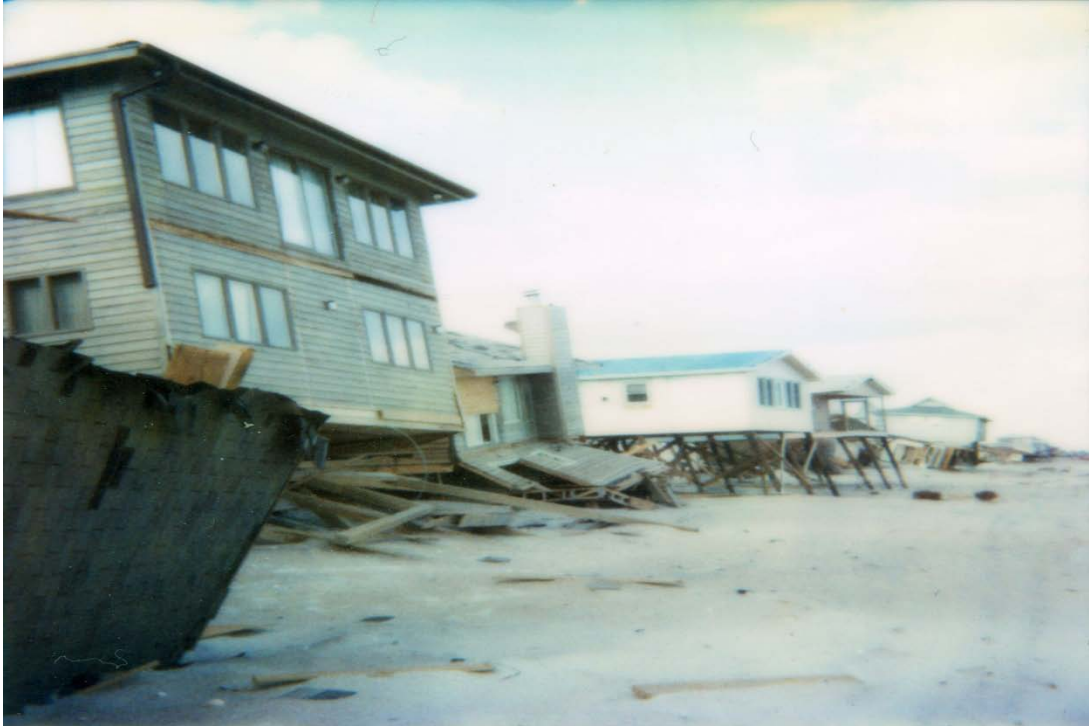
Figure B-10- Coastal storm damage after Hurricane Fran 1996
