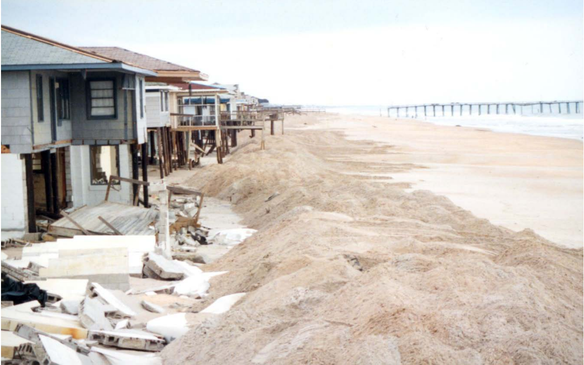
Figure B-4 - Beach scraping following Hurricane Fran
