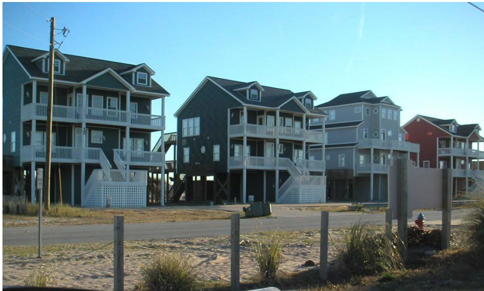
Figure B- 6 - Four typical new structures (all Type 56) built in 2004 on Topsail Island, NC
