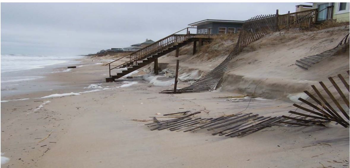
Figure B-5 - Sandbags in place but threatened February 2005.
