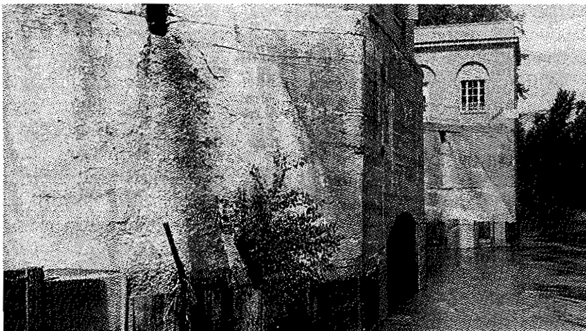
Water Supply Intake.
