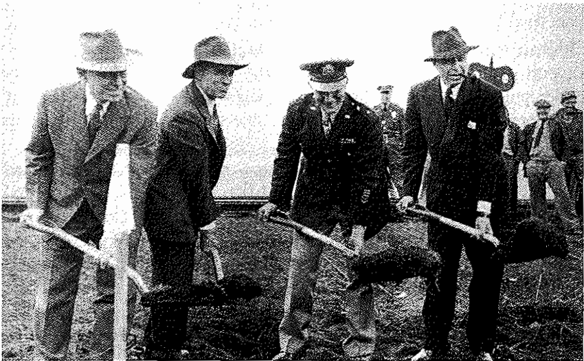
Starting Construction on the Pick-Sloan Plan, 21 March 1946.
