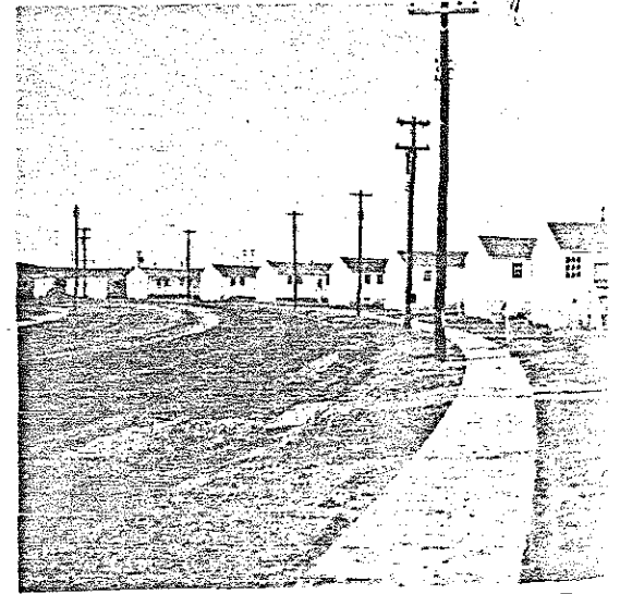
5. Housing at Ft. Randall Dam
