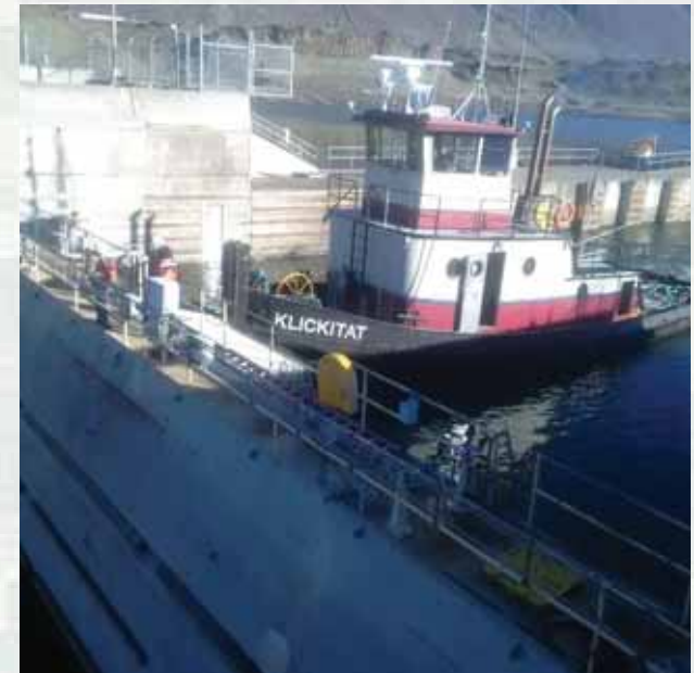
SDS Lumber contract tug moving the floating bulkhead into place at the start of the annual lock maintenance
