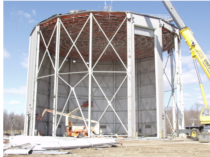
Crews dismantle a reactor facility.
