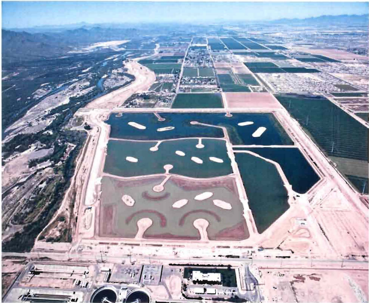
Overall Project View as Constructed features
