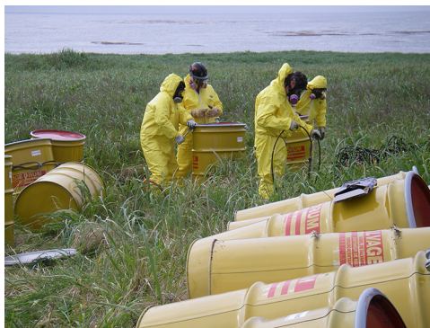
Hazardous waste technicians prepare overpack salvage drums for transportation offsite using helicopter sling loads at Tanaga Island.
