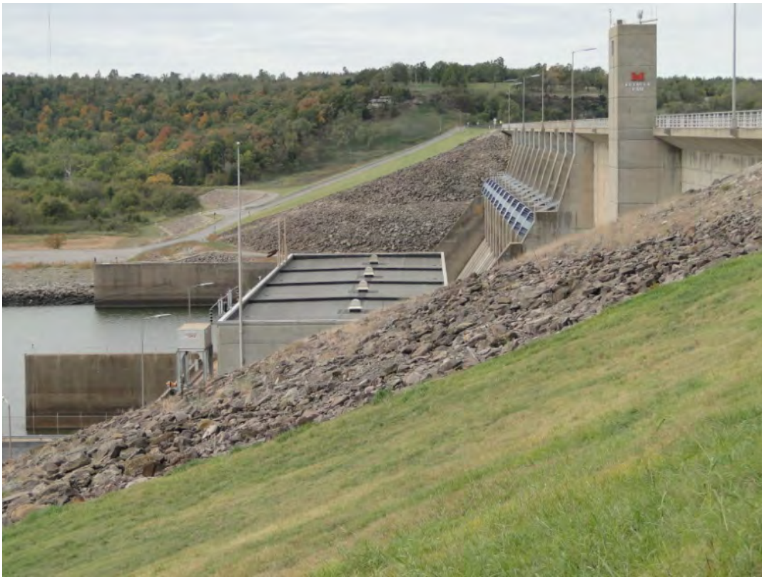
Figure 3.10-3. Prohibited Access Area at Eufaula Dam
