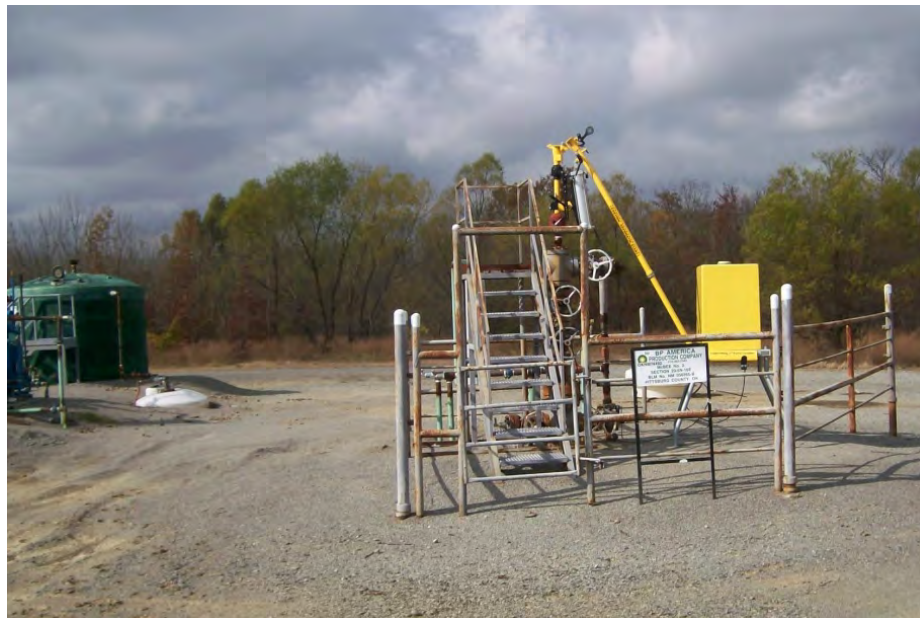
Figure 3.4-2. Natural Gas Well at Eufaula Lake
