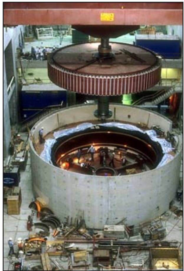
Generator installation at Bonneville Second Powerhouse
