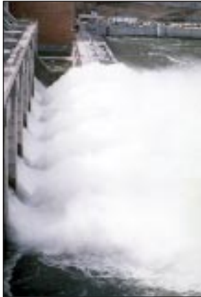
Photo showing Spillway deflectors (flip lips) in operation
