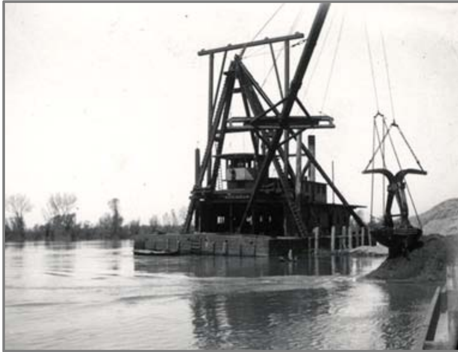
Figure 2-2. Levee Construction in Natomas.
