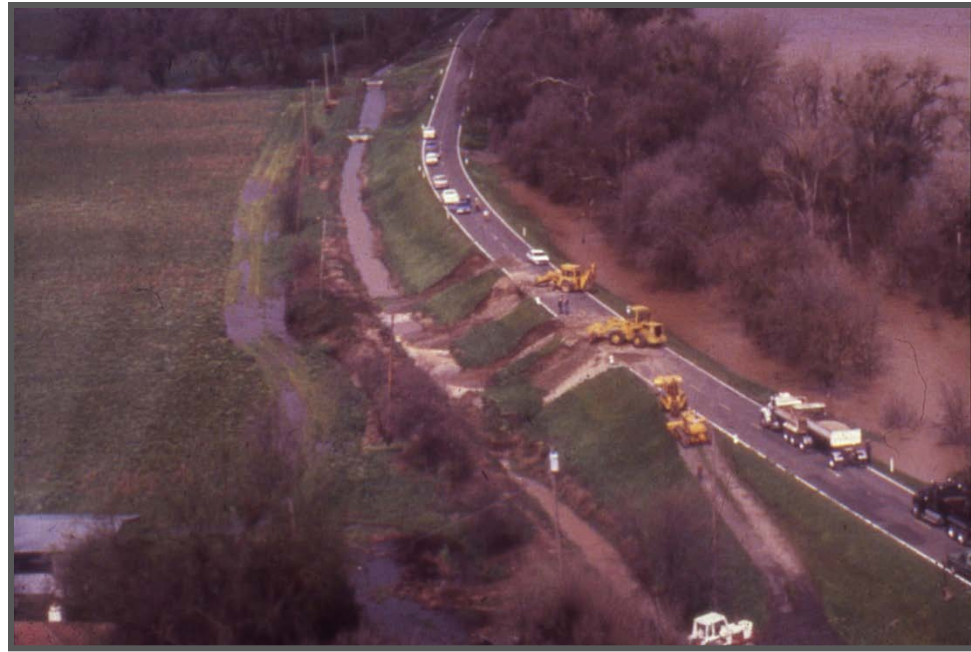
Figure 2-3. Slope Failures on the Landside of the Levee and Seepage Exiting at the Levee Toe on the Garden Highway in Natomas During the 1986 Flood.
