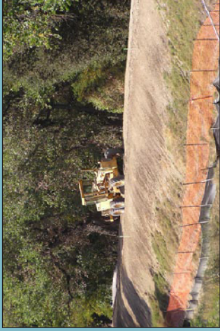
Levee embankment grading
