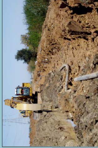
Levee embankment grading
