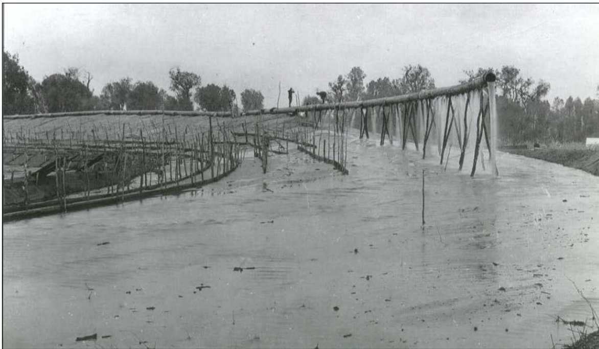
Figure 1-6: Typical Suction Dredge Levee Construction on the Sacramento River System.
