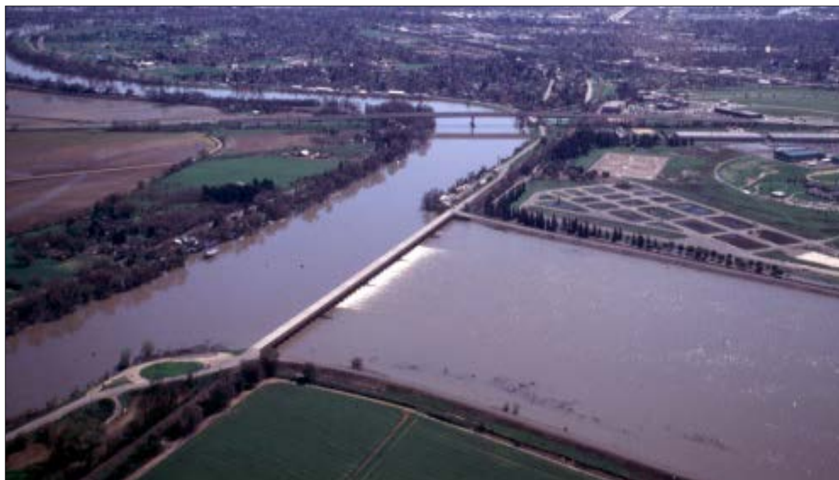
Figure 4-1: Sacramento River overflowing in to the Sacramento Bypass.
