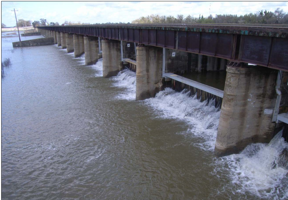
Figure 1-8: The Sacramento Weir.
