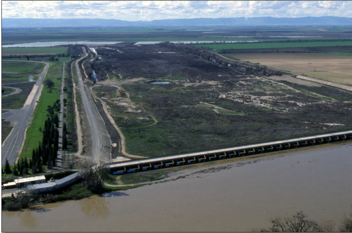
Figure 3-8: Sacramento Weir and Bypass.
