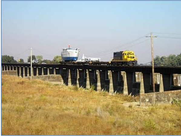
Sierra Northern Railway Bridge crossing over the Sacramento Weir
