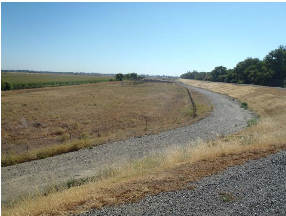
HTRW FIGURE 14 -Old Bryte Landfill adjacent to Sacramento Bypass (7) north levee.
