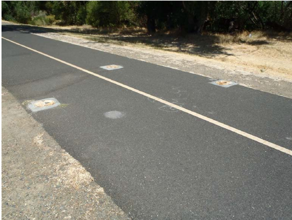
HTRW FIGURE 13 - ARS Reach C Monitoring well cluster in the levee crown near Martin Sprocket & Gear
