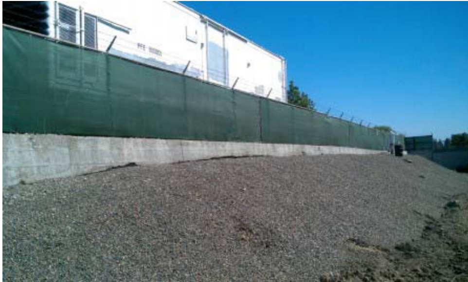
HTRW FIGURE 19 -ARS Reach D (6) This former PG&E manufactured gas plant site is currently under remediation. Contamination has been solidified in place at the foot of the levee. Remediation is planned to be completed in November 2012. Active railroad tracks are also present on top of the levee in this area.
