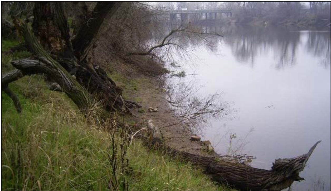
Figure 1-3. Erosion site on left bank near LAR RM 0.3 (2008)
