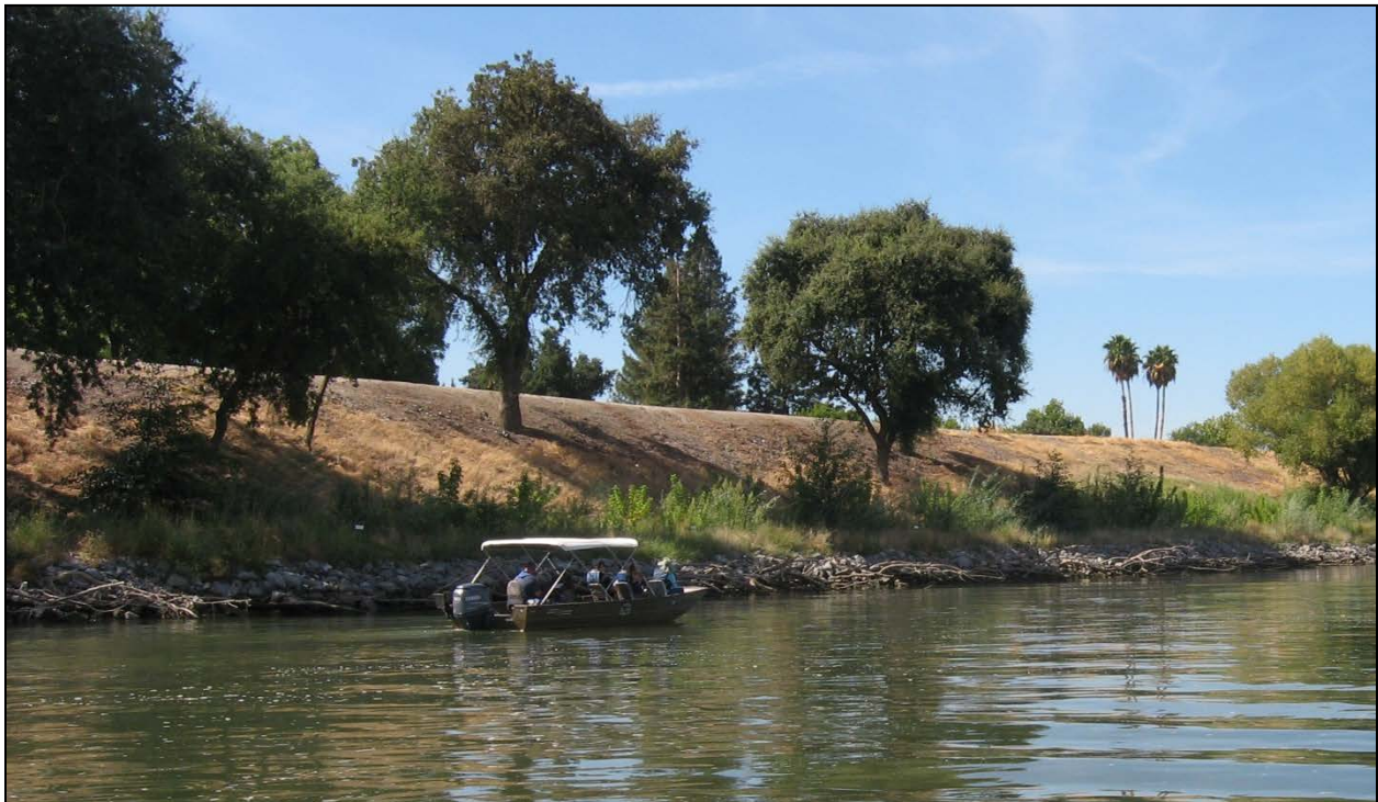
Figure 2-7. Repaired site at Sacramento River left bank RM 53.2 (2009)
