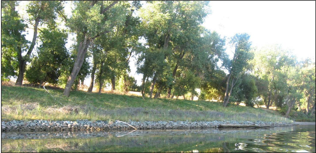
Figure 2-2. View of repair site on the left bankline near LAR RM 0.3 (2009)
