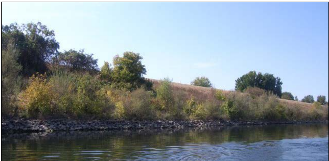
Figure 2-3. View of repair site on left bankline near LAR RM 4.3 (2010)
