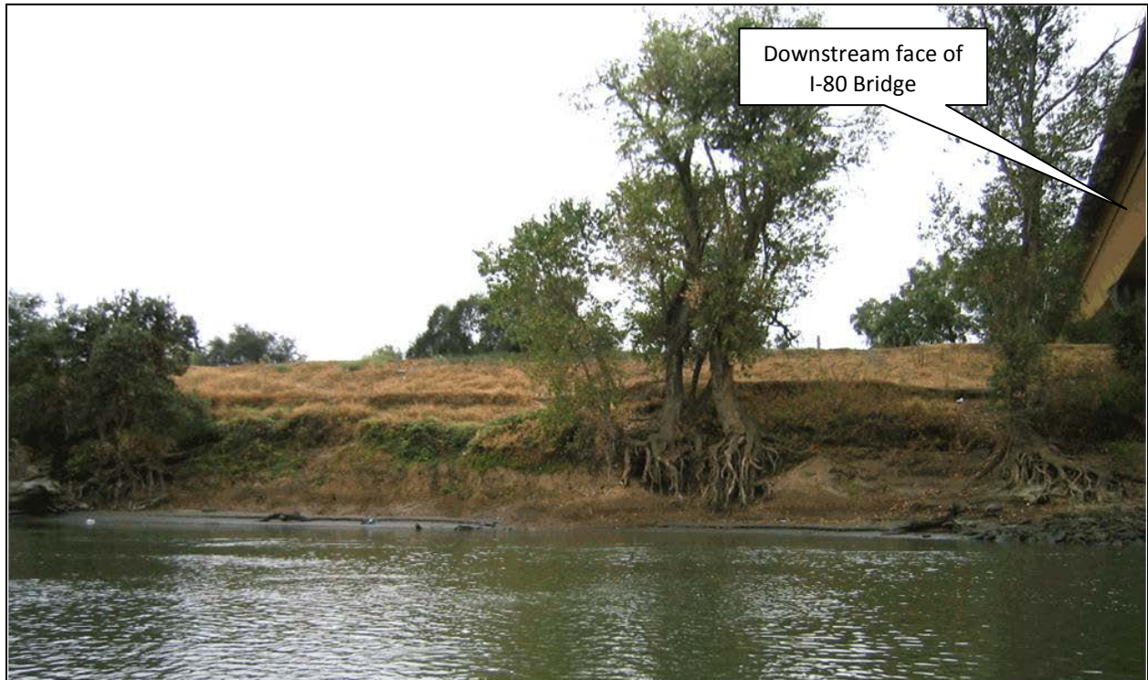
Figure 2-4. Erosion site of the right bank of the Sacramento River at RM 62.5 (2005)
