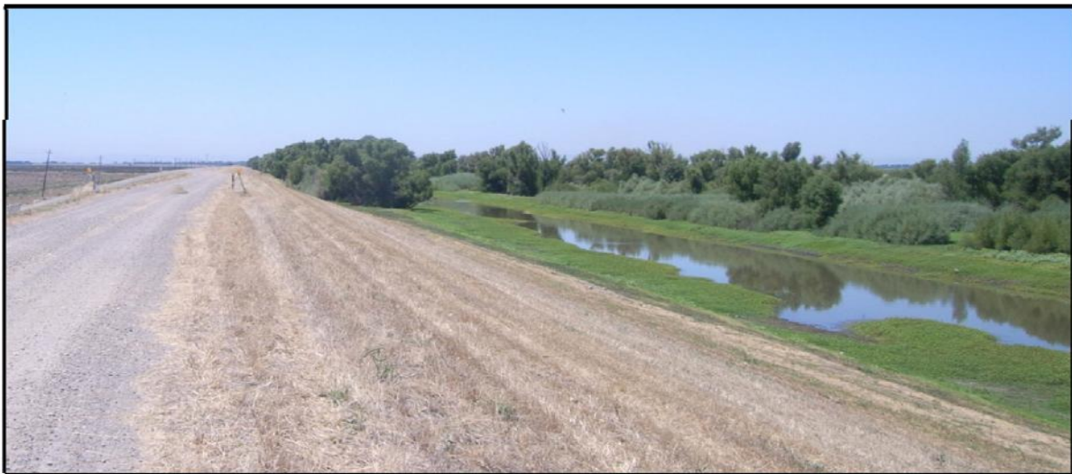
Figure 8-5. Typical View of the Natomas Cross Canal
