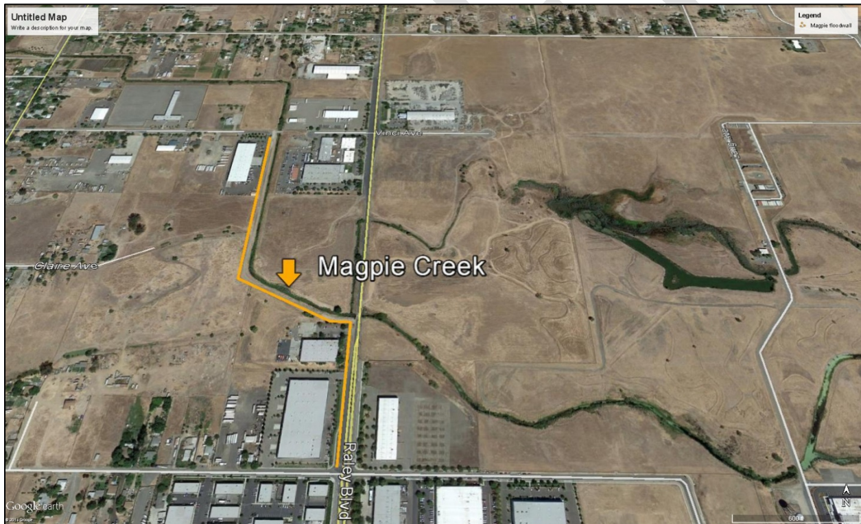
Figure 10. Floodwall and New Levee along Magpie Creek.
