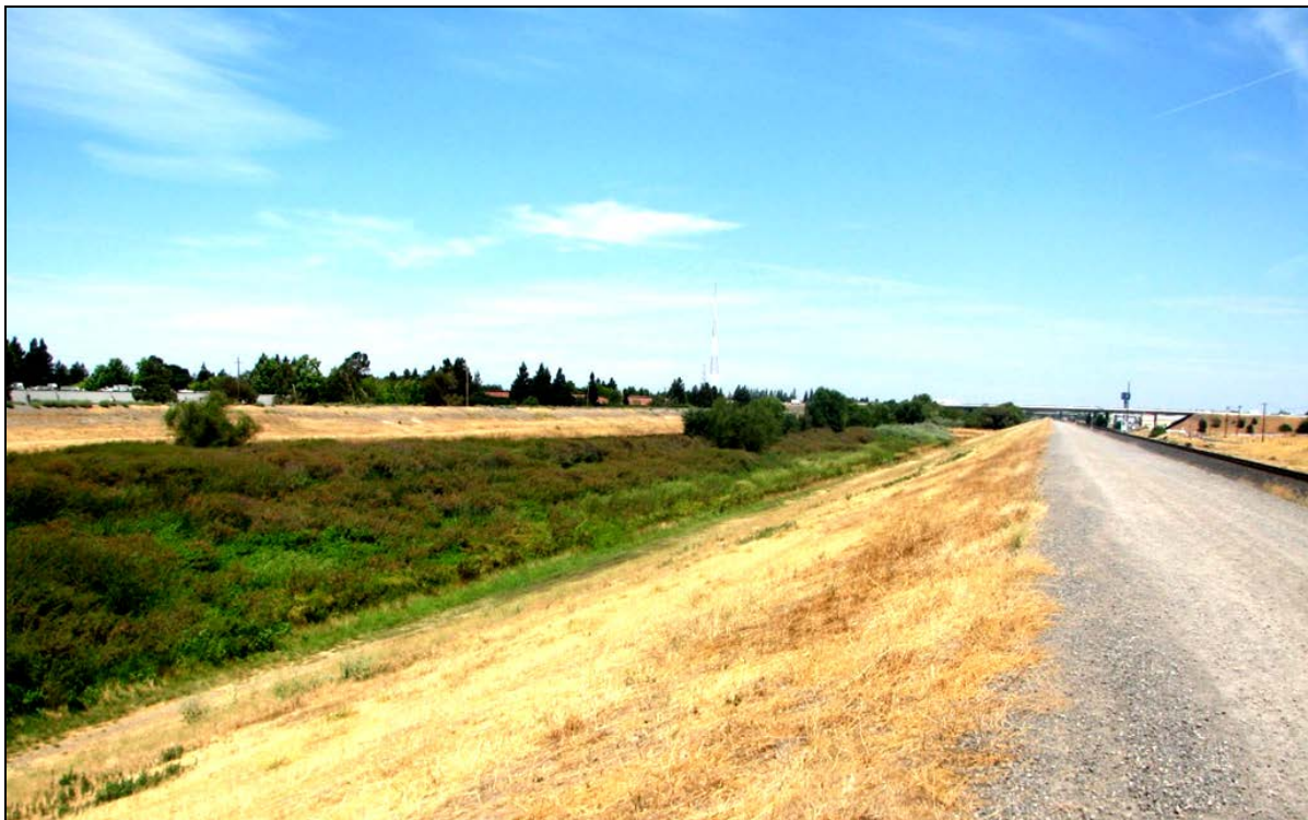
Figure 19. Natomas East Main Drain Canal.
