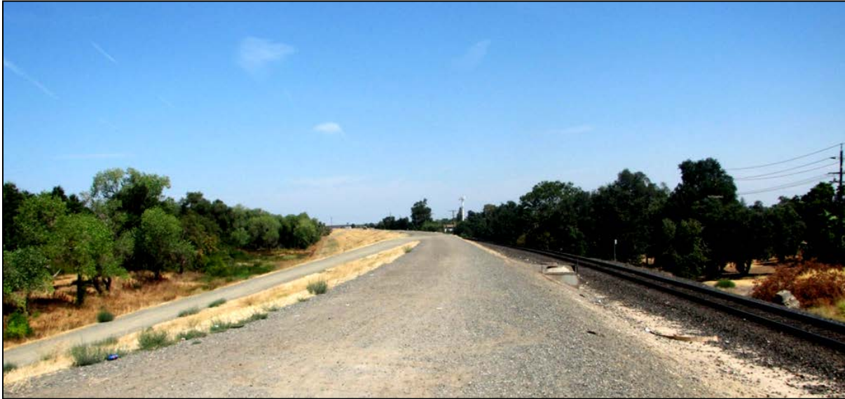
Figure 20. Natomas East Main Drain Canal Levee.
