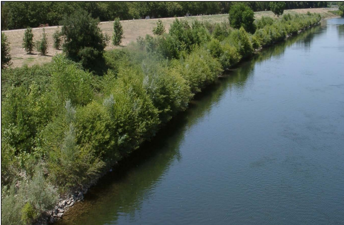
Figure 9. Planting Site 4L on the American River after Bank Protection in 2005.
