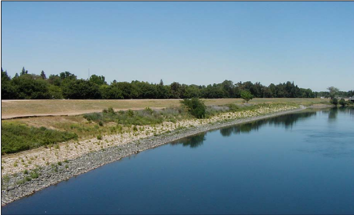
Figure 8. Planting Site 4L on the American River after Bank Protection in 2001.
