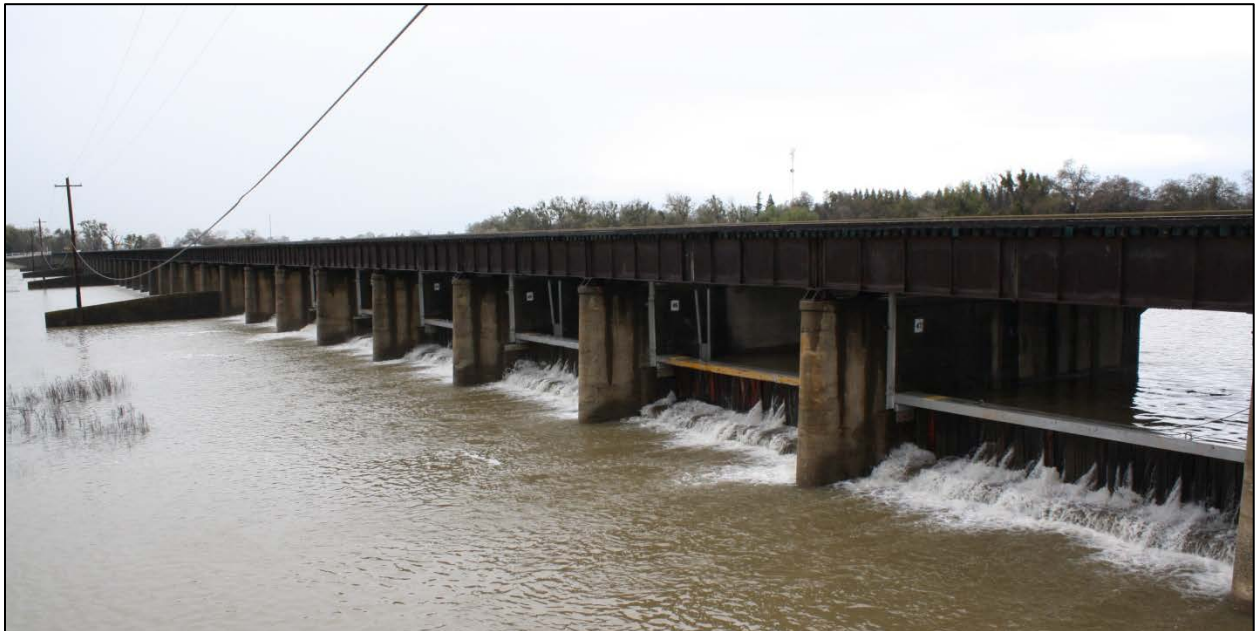
Figure 27. Sacramento Weir in High Water Event.
