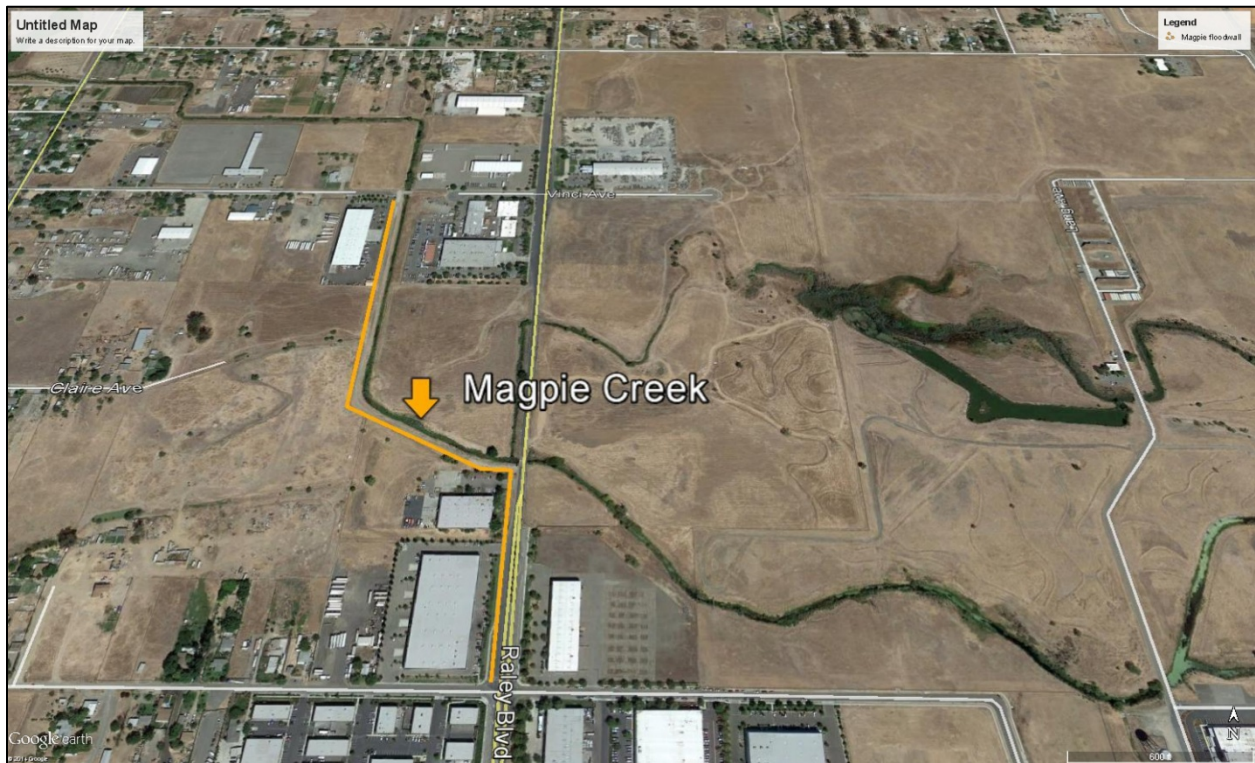
Figure 6. Floodwall and New Levee along Magpie Creek.
