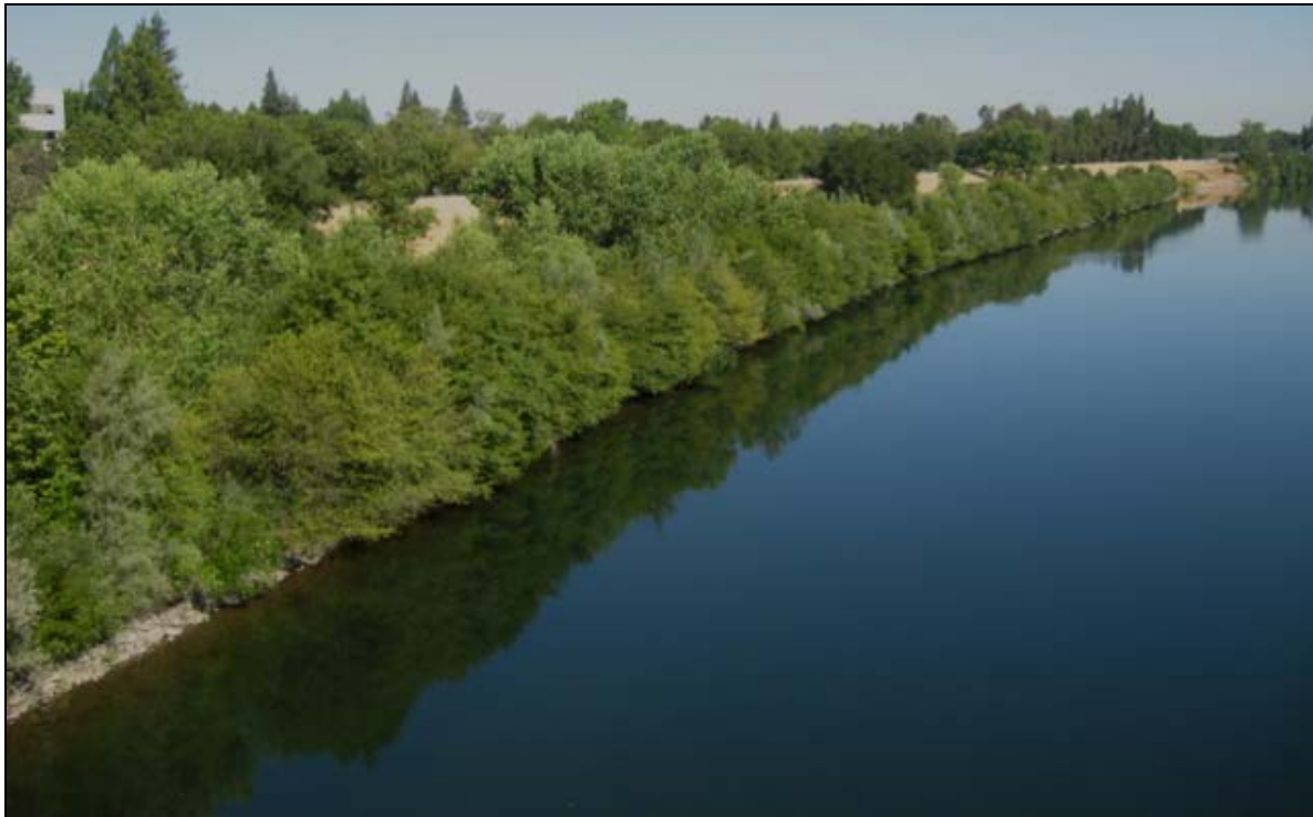
Figure 10. Planting Site 4L on the American River after Bank Protection in 2010.
