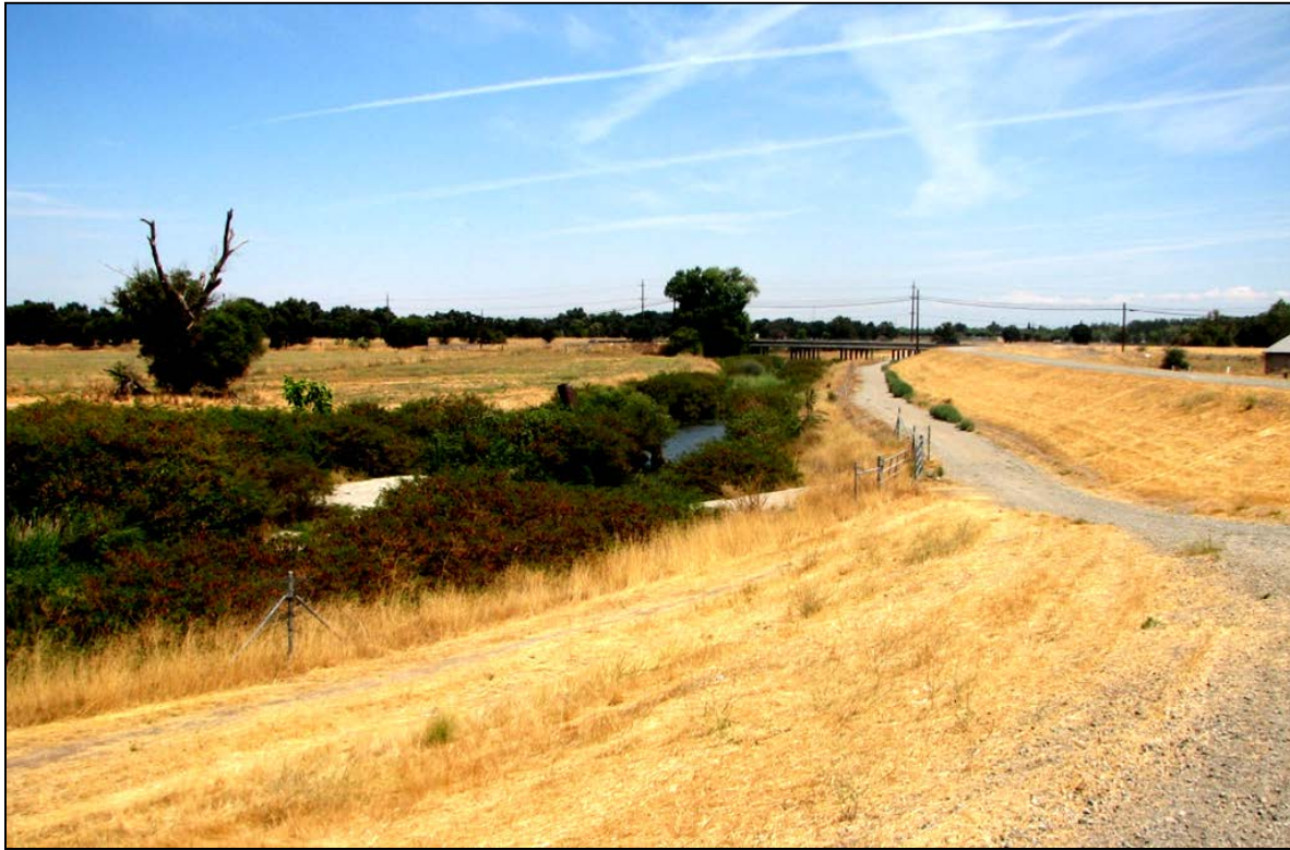
Figure 23. Dry/Robla Creek Levee and Channel.
