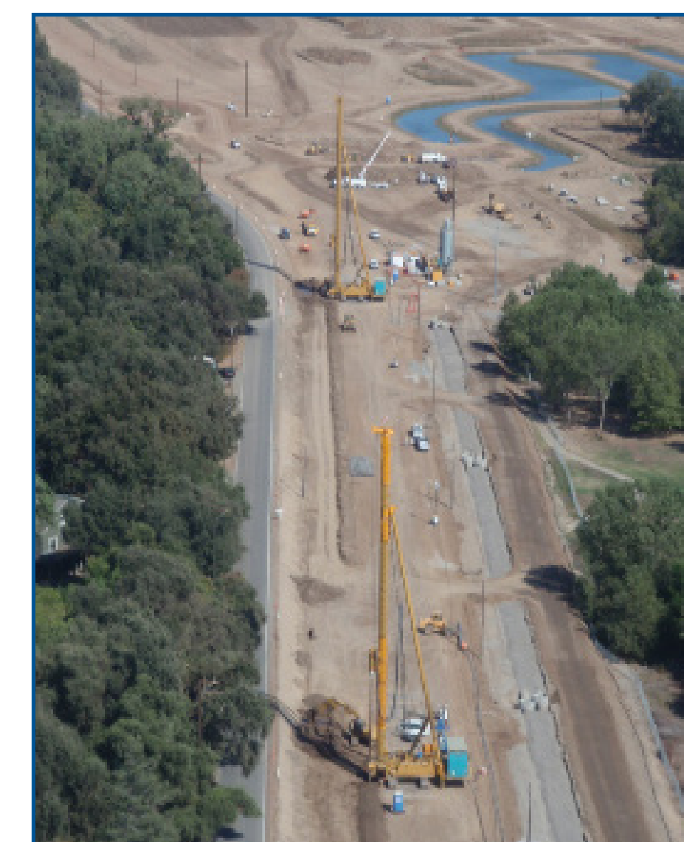
BELOW: Levee instability repair
