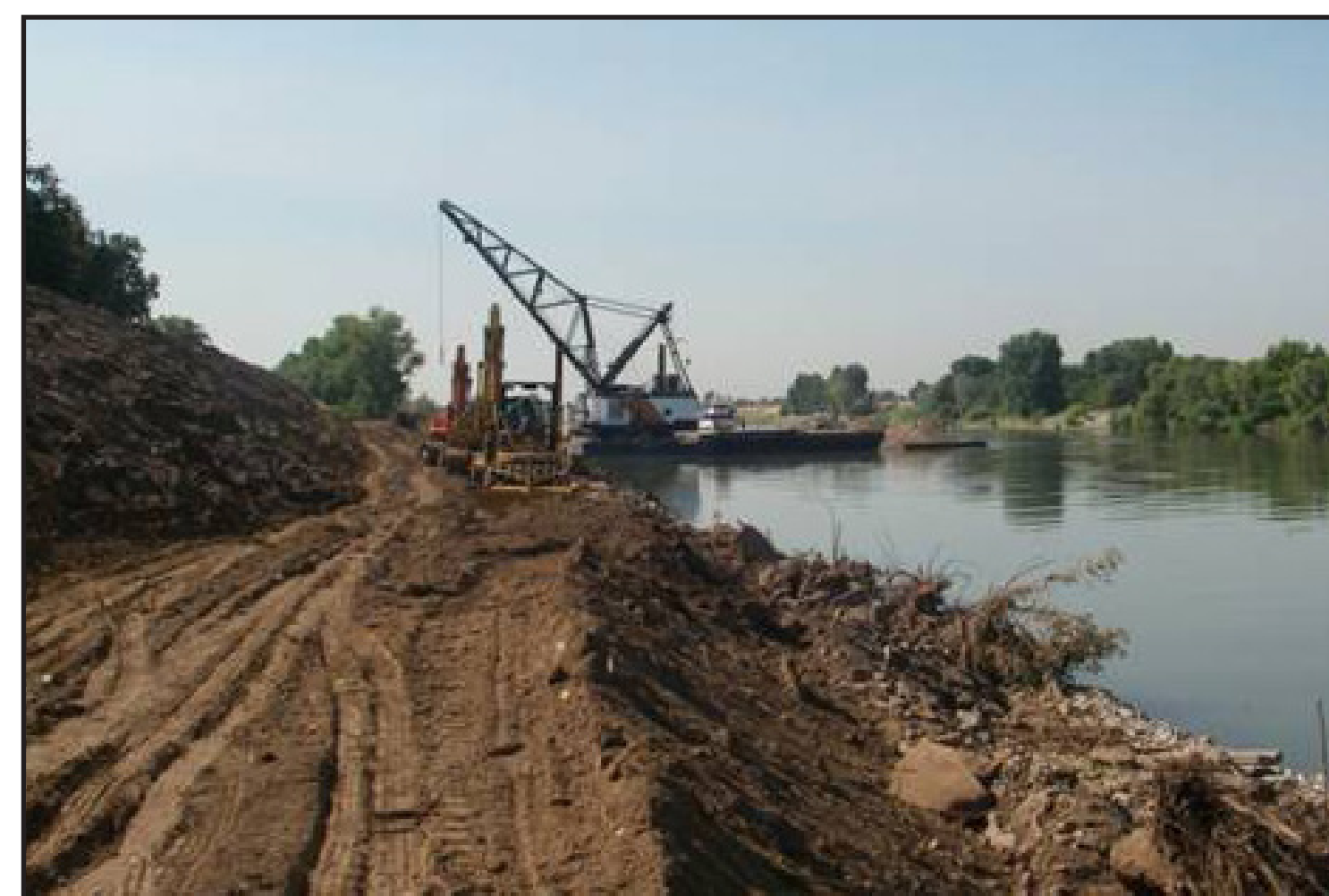
Typical bank protection placing rock riprap revetment from barge
