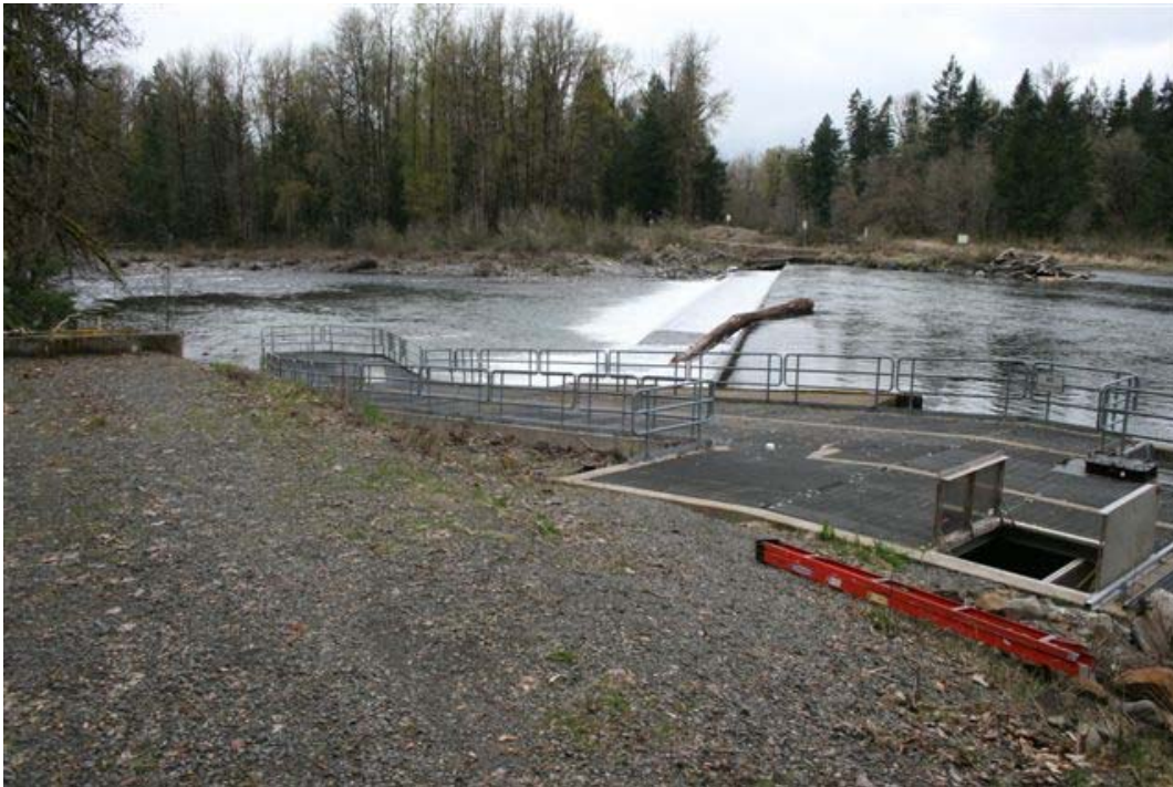
Figure 3. Existing Fish Ladder and Trapping Facility at Upper Bennett Dam.
