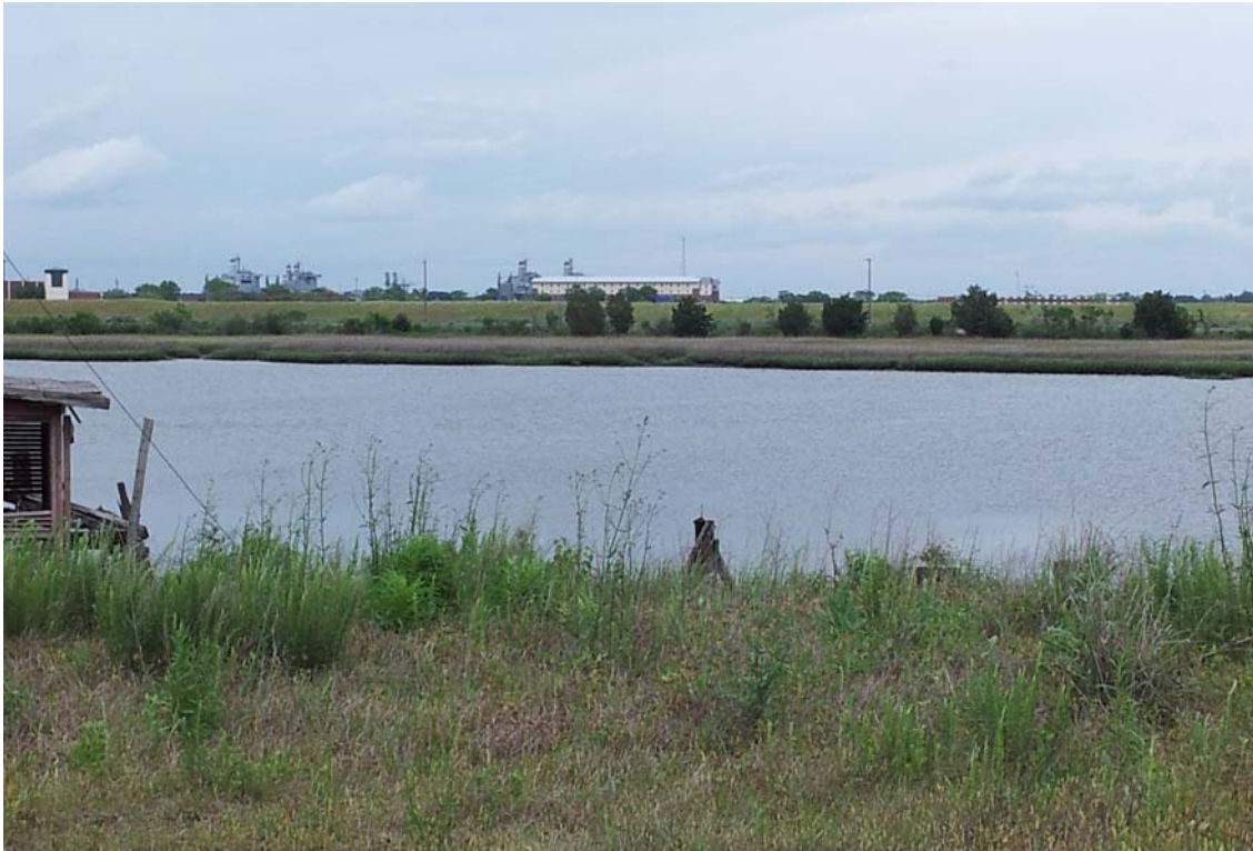
Photo 8 -- Proposed wharf area (south portion) on Shipyard Creek
