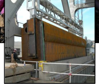
A RSW is towed upriver for installation at Lower Monumental Lock and Dam (above); a TSW is lowered into a spillbay at McNary Lock and Dam (right).
