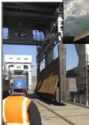
Temporary spillway weirs were installed at McNary Lock and Dam, near Umatilla, Ore., John Day Lock and Dam, near Rufus, Ore., and Little Goose Lock and Dam, near Starbuck, Wash.
