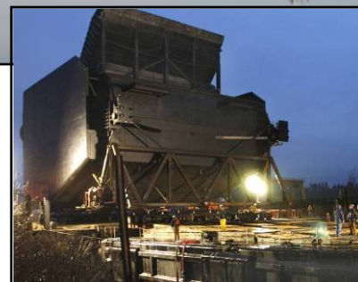
A removable spillway weir was installed in February 2005 at Ice Harbor Lock and Dam, near Burbank, Wash.
