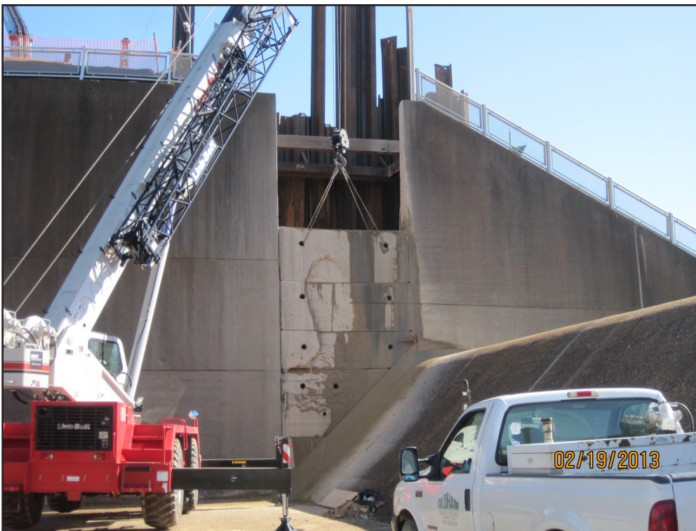
Concrete being removed at Sardis Lake Spillway.
