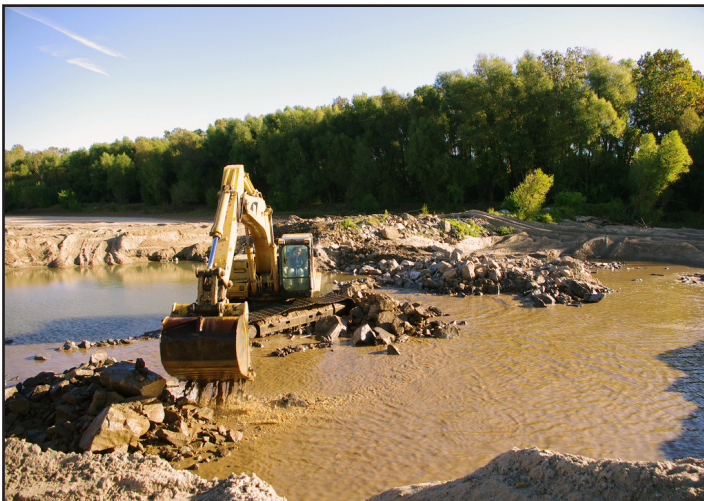
The above photo show a dike notch being constructed and the below photo shows the constructed dike notch.
