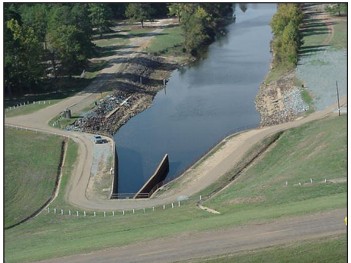
Bayou Bodcau Dam and Reservoir
