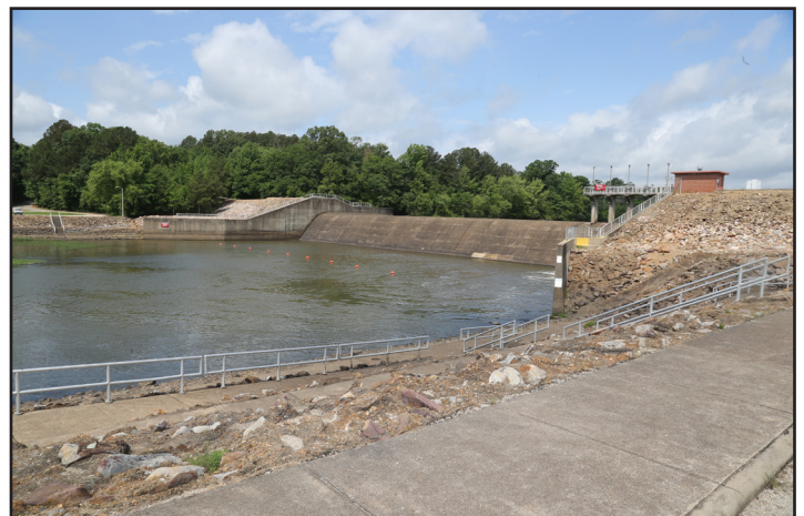
Re-regulation Dam at DeGray Lake
