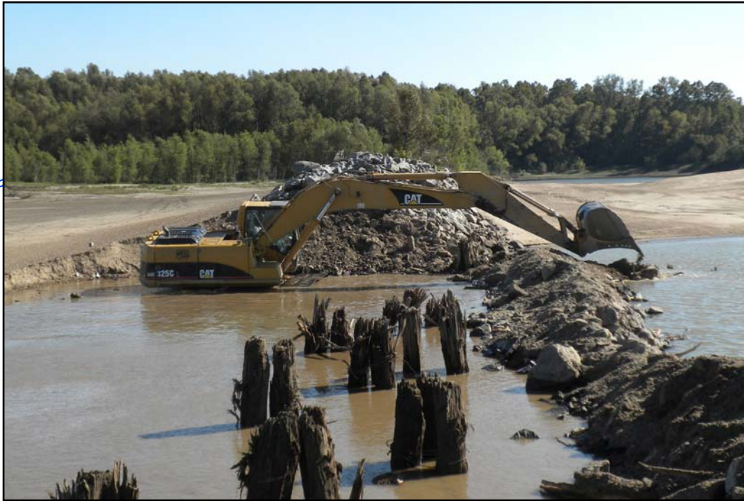
Timber piles that were placed in 1963 are being removed at dike 2.
