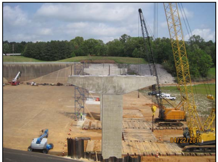
Construction of bridge piers in April 2011.
