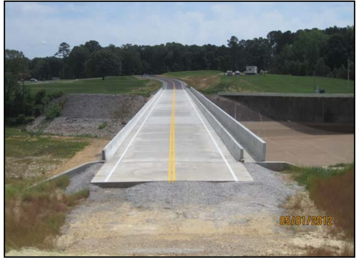
Completed bridge with south approach road.
