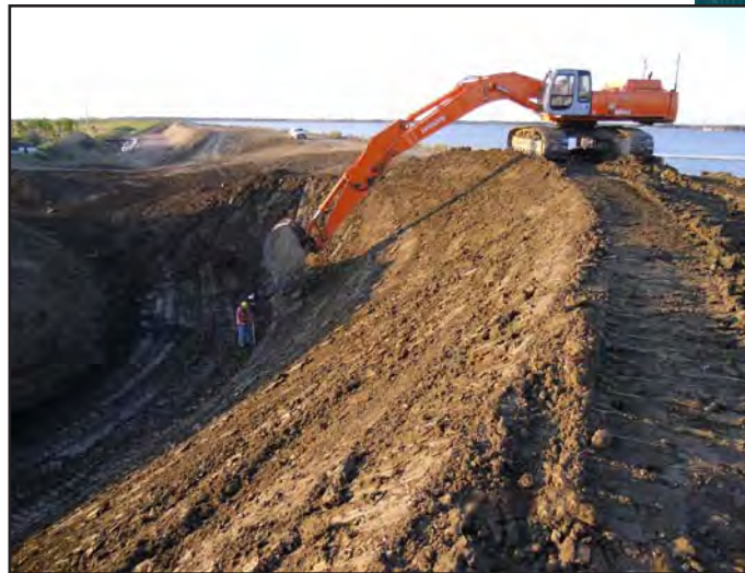
Work being done on the Louisiana levee side.
