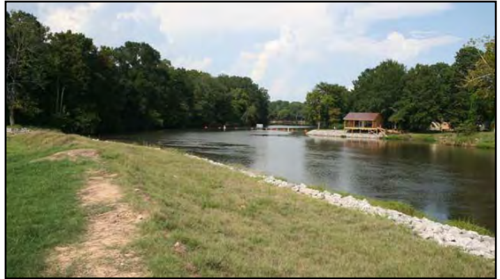
Standing on the east bank of the Little Tallahatchie River looking toward the Sardis Lower Lake.
