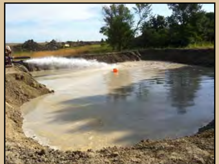
Worker adds bentonite to slurry pond with water pump.
