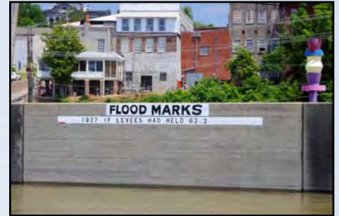
Flood water at city front, Vicksburg, covers all previous flood mark levels.
