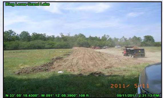
Ring levee being built at Grand Lake berm.
