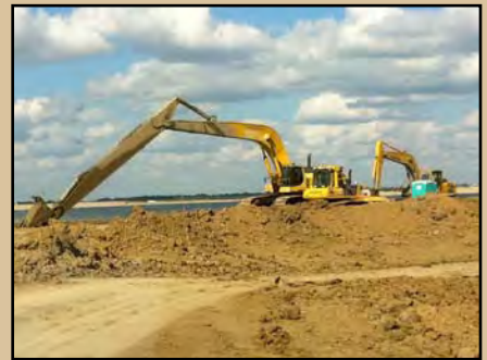
Slurry trench construction at Devils Lake.
