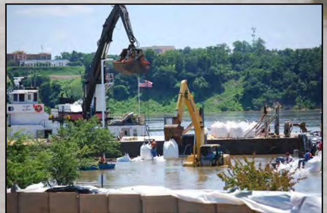
Sandbags being placed at Natchez Under the Hill
