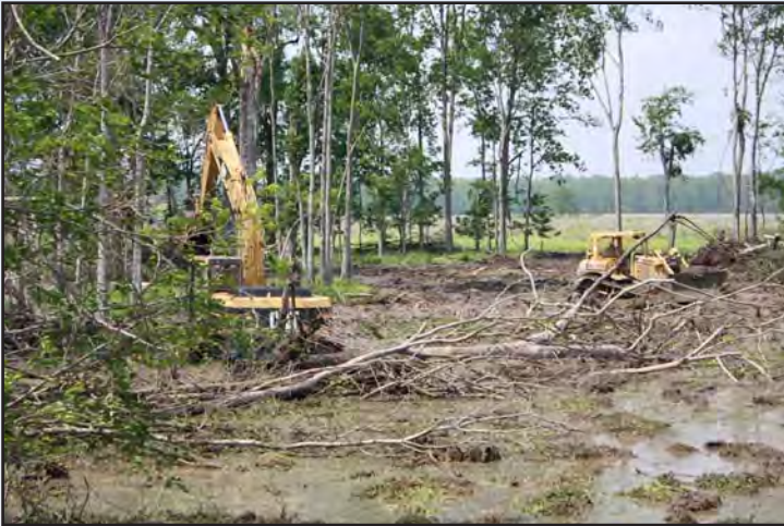
Work at Buck Chute.
