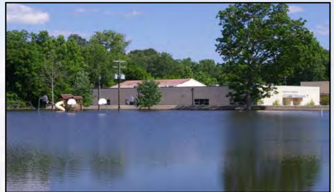
Levee protects Redwood Elementary School from flood water.
