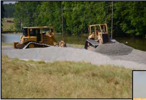
Albermarle levee slide stabilization
