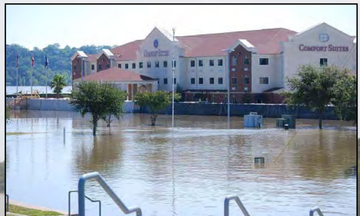
Flood waters surround the Comfort Suites Hotel at Lake Village, Arkansas.
