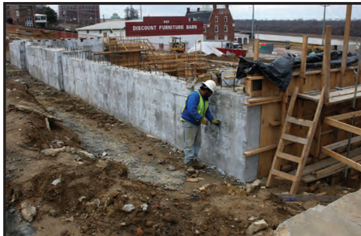
A contractor works on the wall of the museum.
