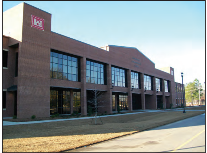
Environmental Laboratory at ERDC.
