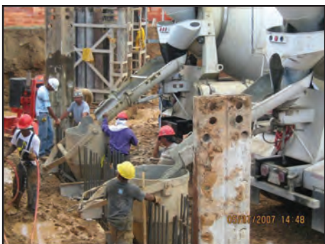
Workers pour concrete into the wall
