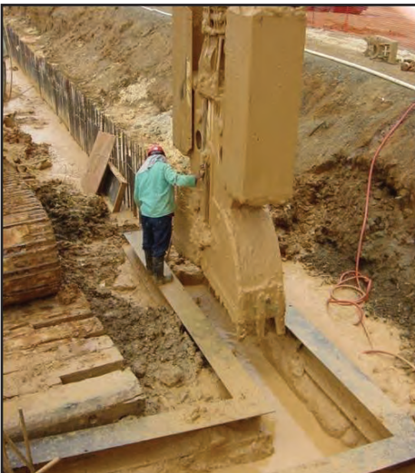
Excavating the trench, filling it with slurry
