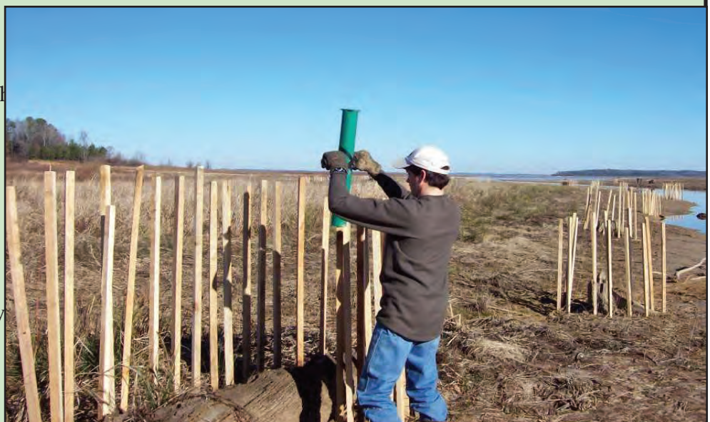
Rob Hoff places stakes at Grenada Lake for fish habitat.
